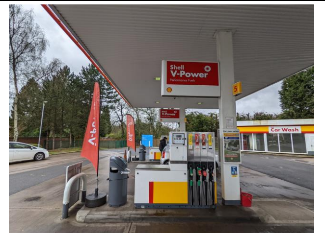
D View of pumps and car wash to the south
