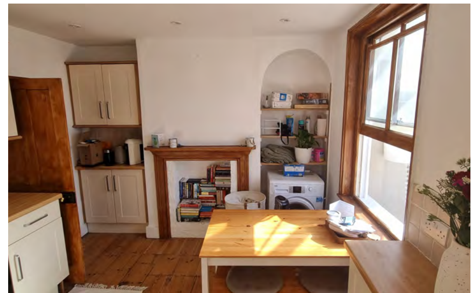
Kitchen showing altered fireplace
