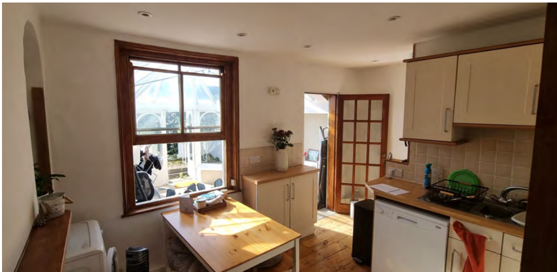
Kitchen showing modern partition and replacement rear joinery
