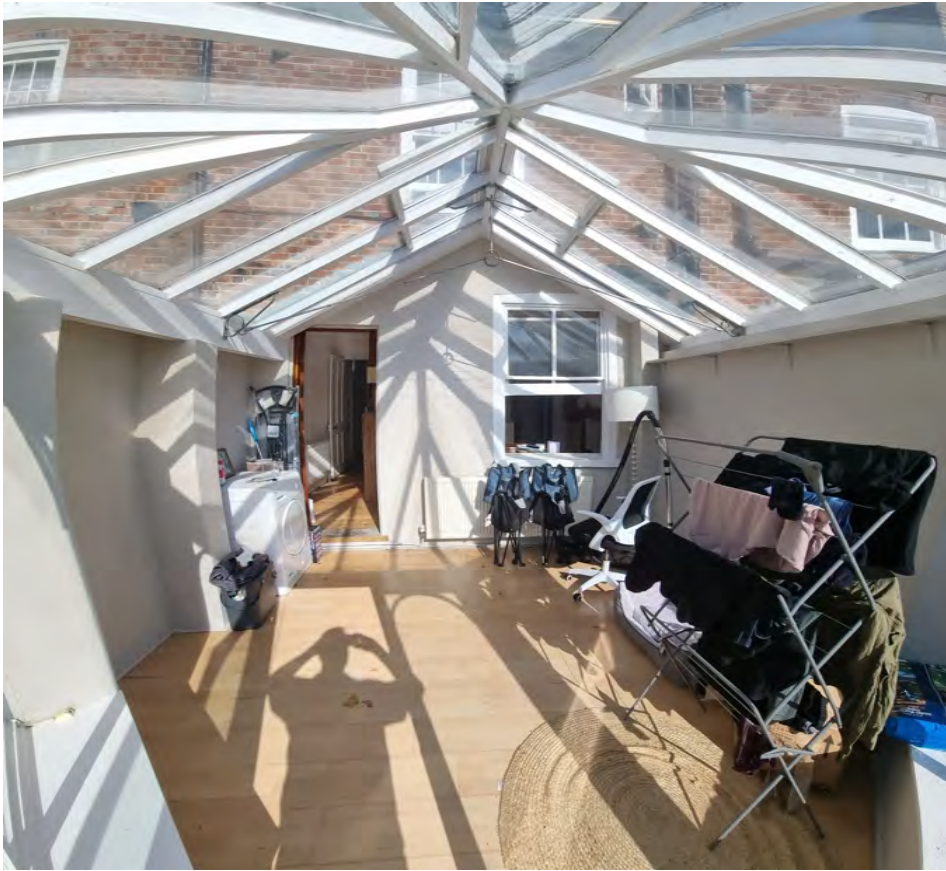
Conservatory looking towards rear of house
