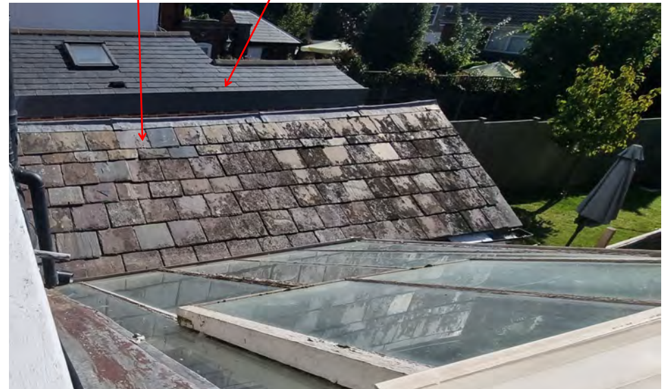
Rear outshot to no. 15 and 14 to the east
