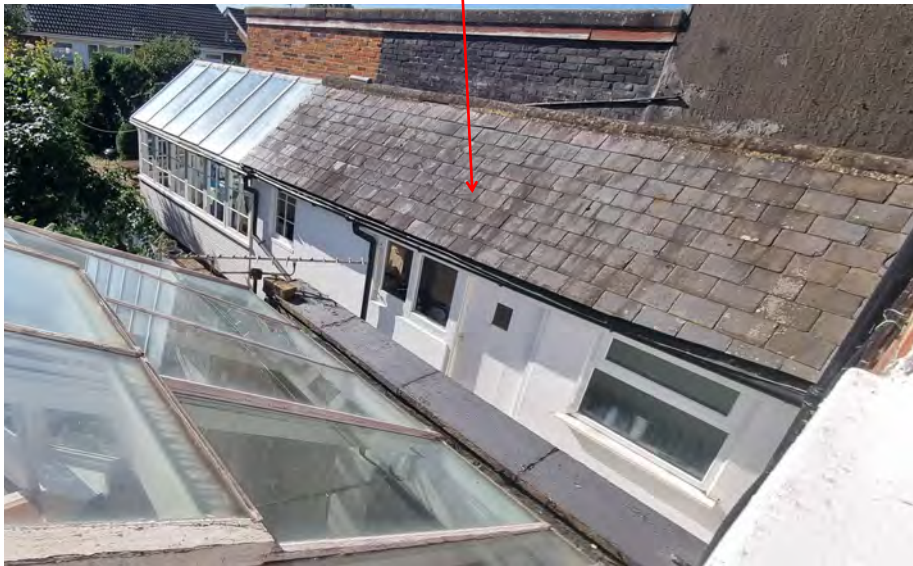
Extended rear outshot to no. 17 to the west
