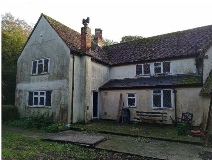
Fig 29. Existing single storey extension to be demolished.
