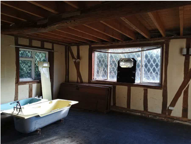
Fig 17. 1964 Extension. Faux Oak timbers within wall.
