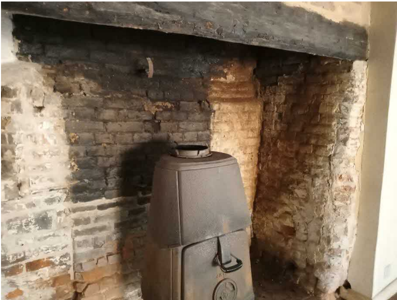
Fig 10. West bay of 17 th century fireplace
