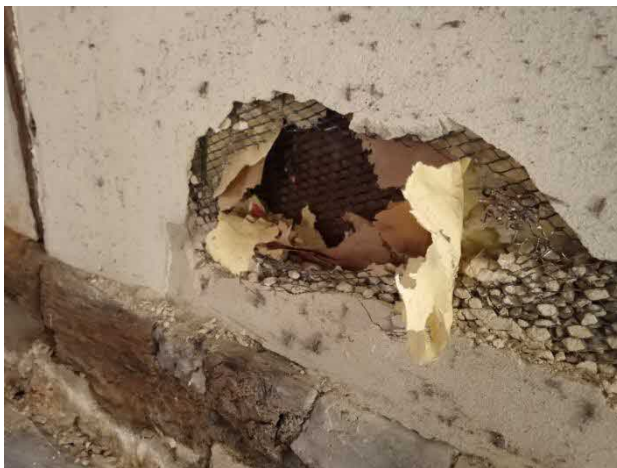
Fig 27. View of external wall within 17 th century building showing plaster on EML both internally and externally
