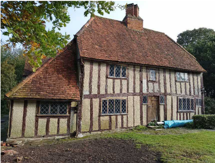
Fig 1. South elevation (original 17 th century building)
