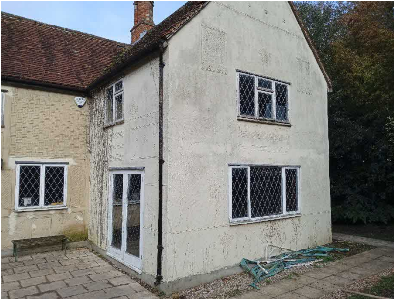
Fig 7. East elevation (later 1964 extension gable)
