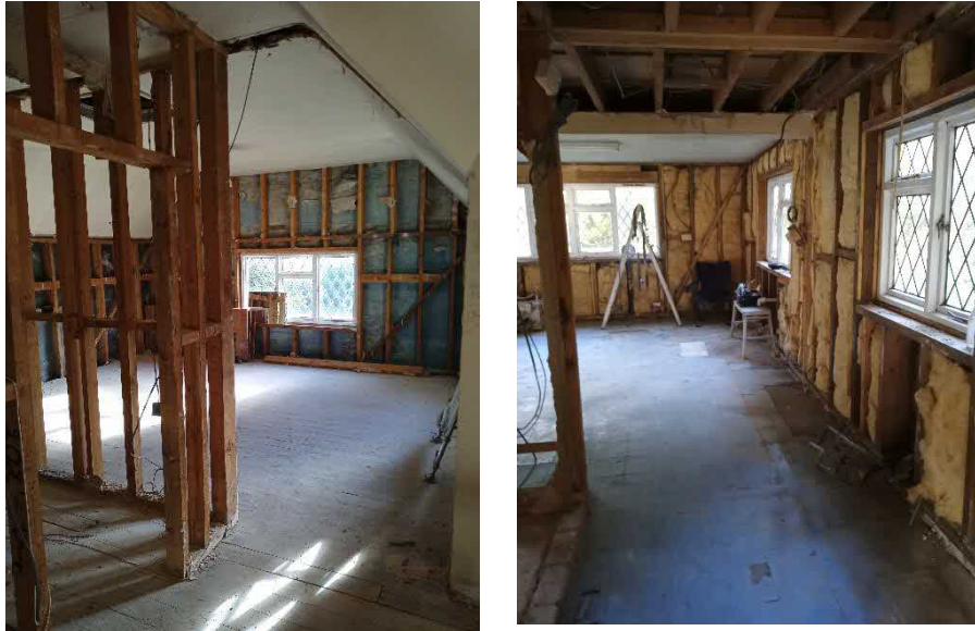
Fig 33. 1 st floor external walls within 1960's extension.
