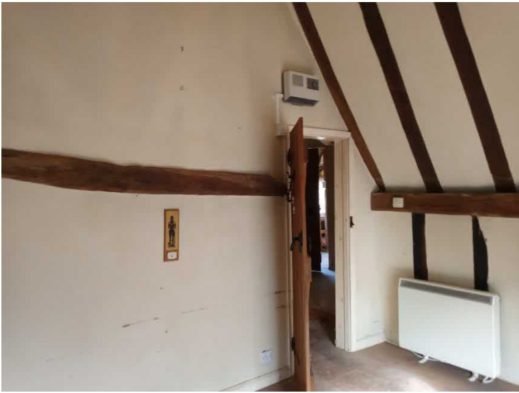
Fig 13. East bay, 1 st floor of 17 th century building
