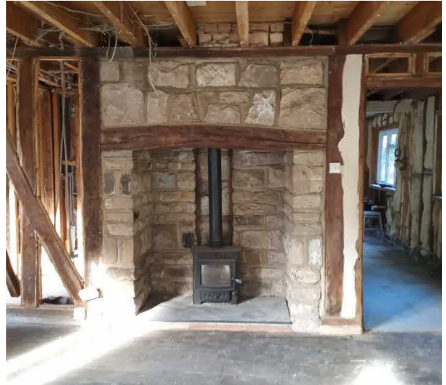
Fig 31. Faux fireplace to be removed
