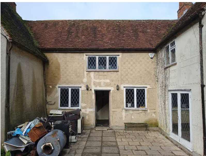
Fig 6. East elevation (later 1964 extension forming an H shape courtyard and new front door facing East)
