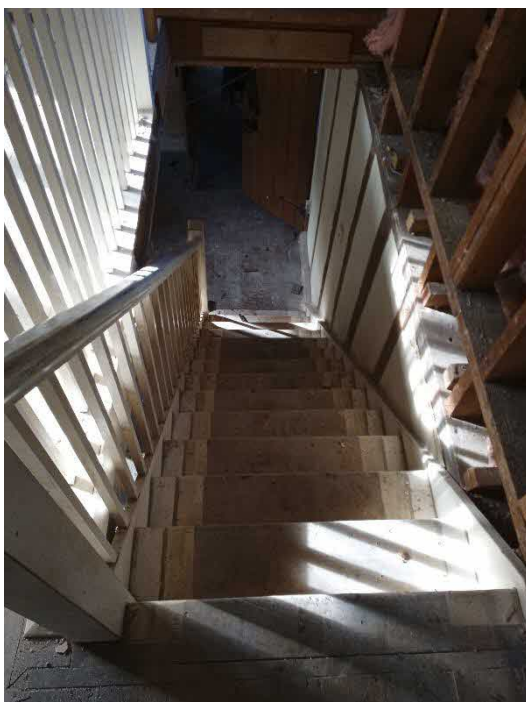
Fig 30. Existing 1960's staircase to be demolished.
