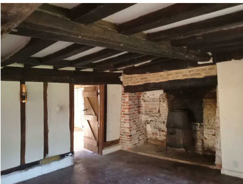
Fig 9. Internal view of West bay of 17 th century building
