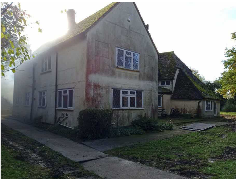
Fig 4. West elevation (Later 1964 extension)
