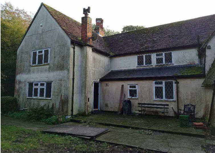
Fig 3. West elevation (Later 1964 extension)
