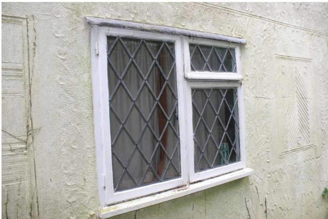
Detail of one of the 1964 casement leaded light windows.
