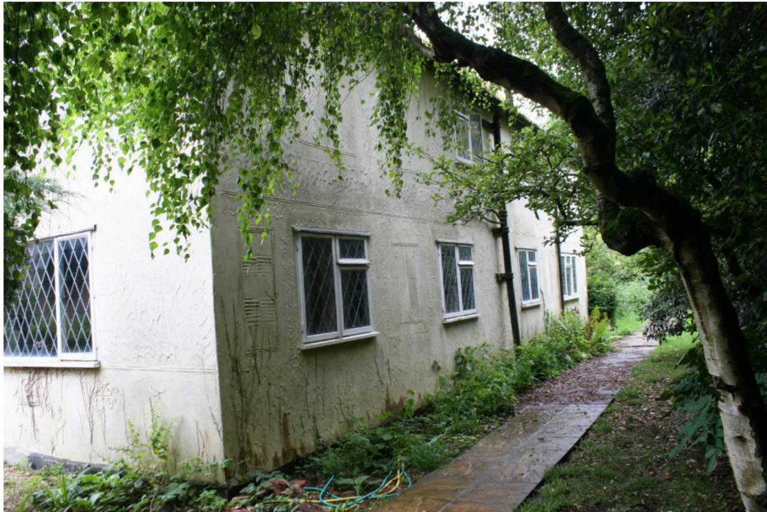
The north elevation looking W.
