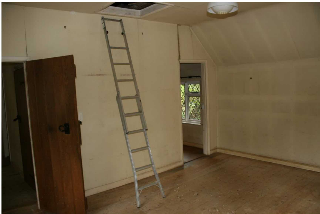
Looking NW in the NE Bedroom.
