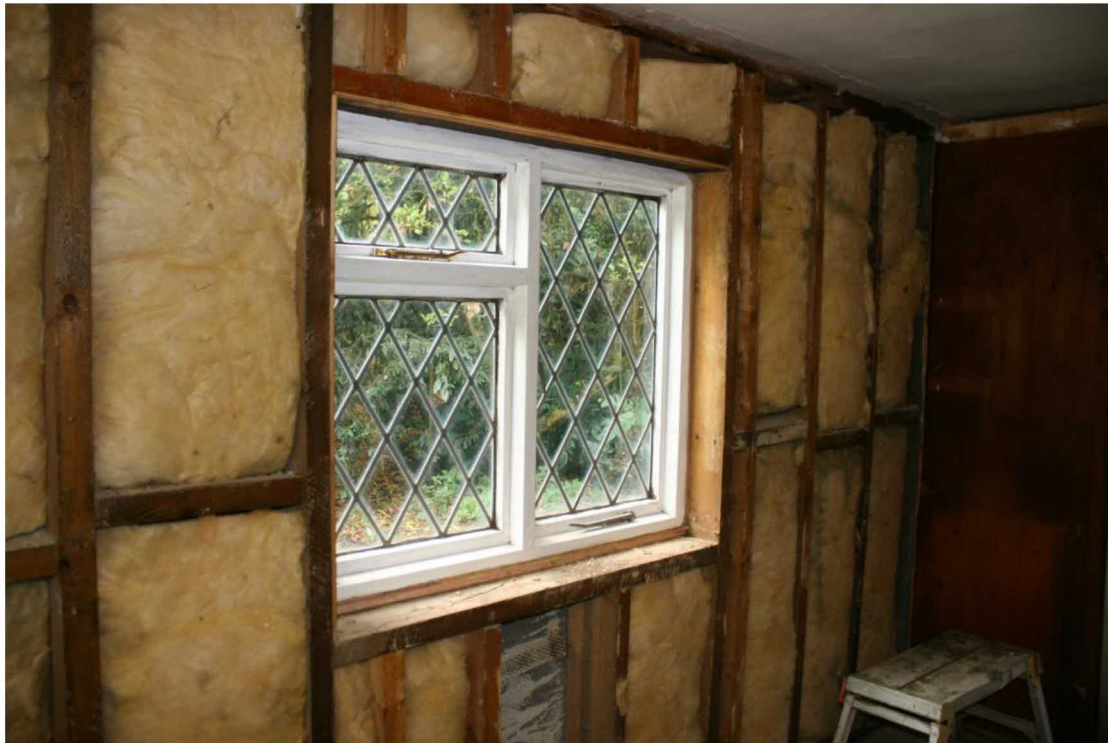
Detail of the wall construction and the leaded light windows.
