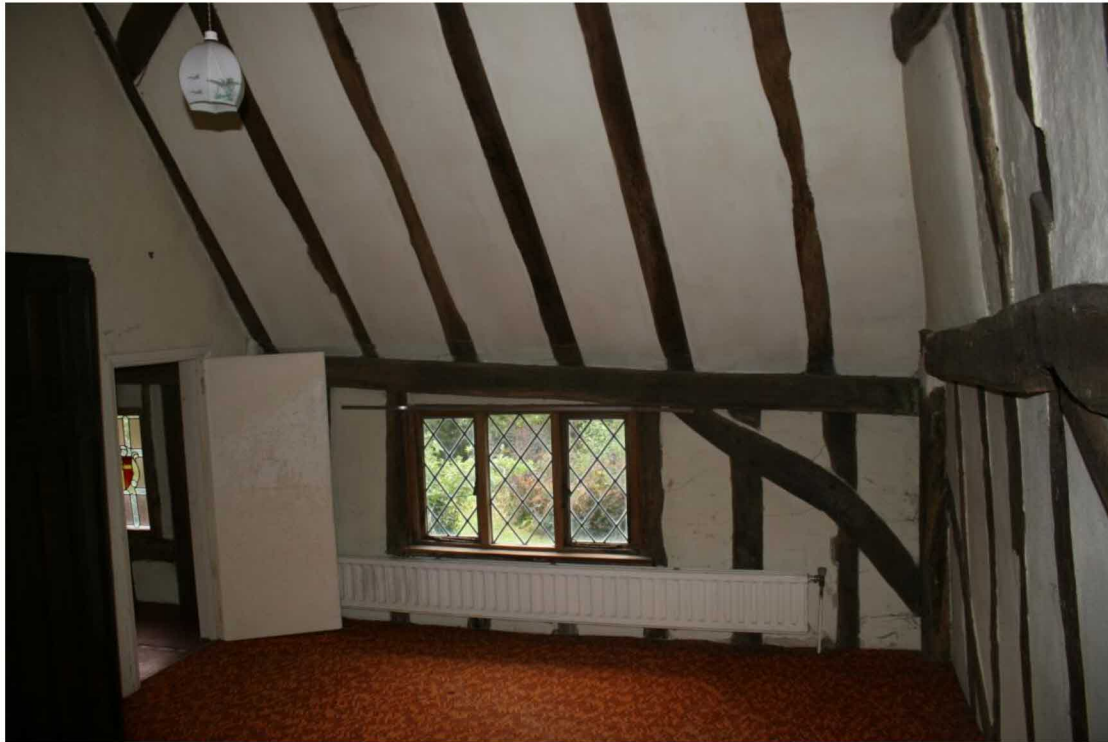
Looking S in the SW Bedroom.
