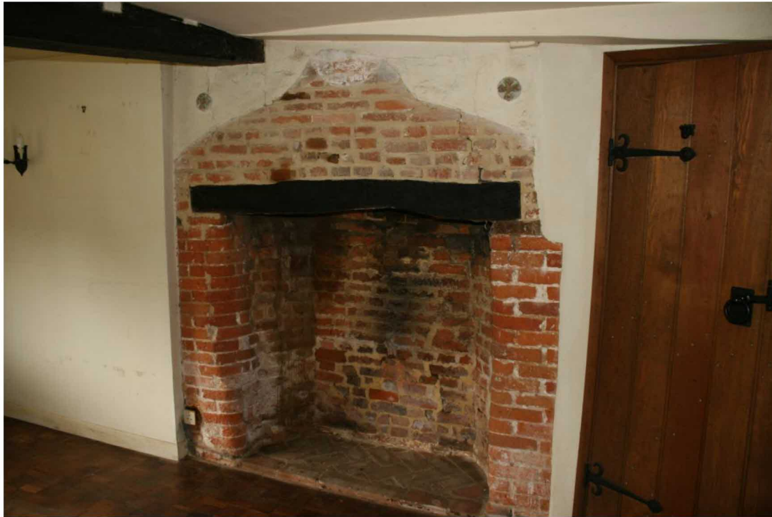
Looking W at the central firestack.
