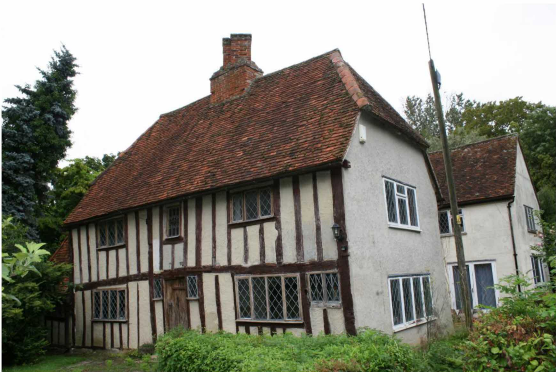
The exposed frame of the south elevation.
