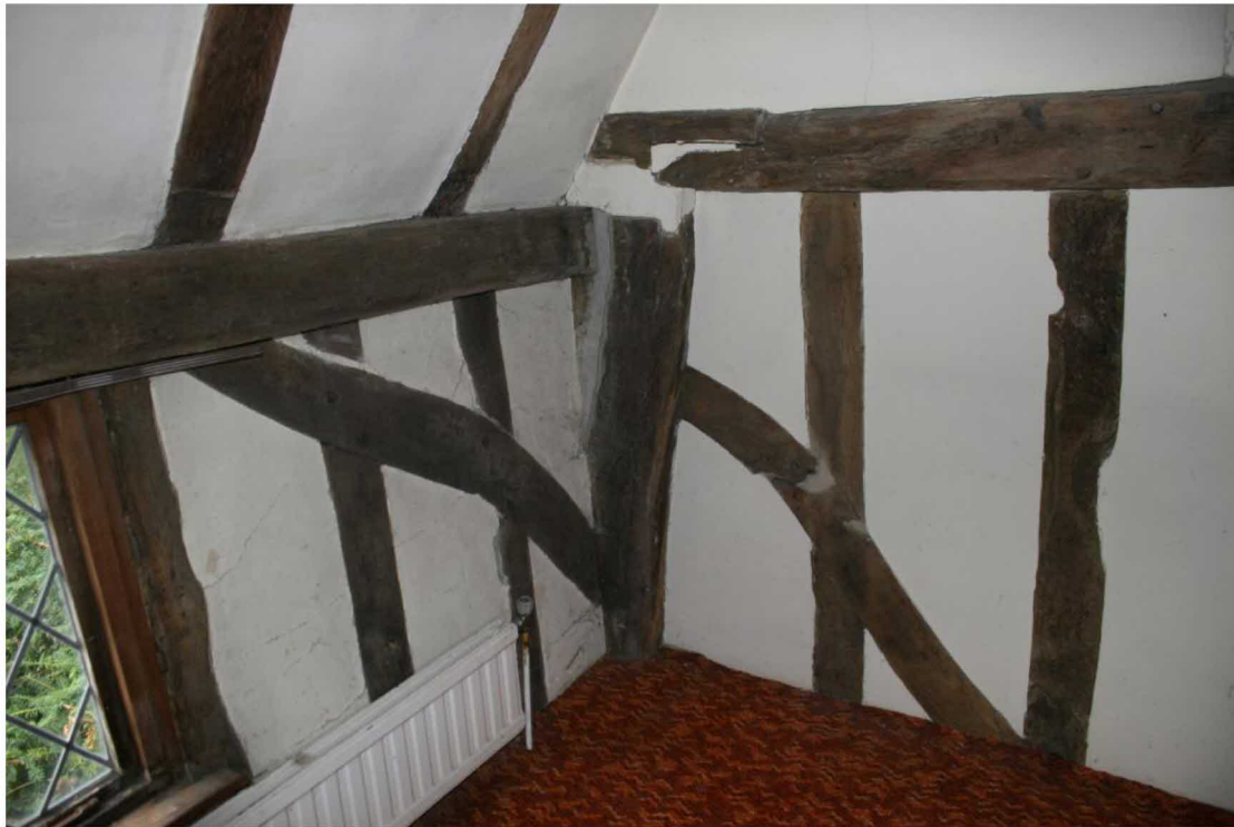
The racked frame in the SW corner.
