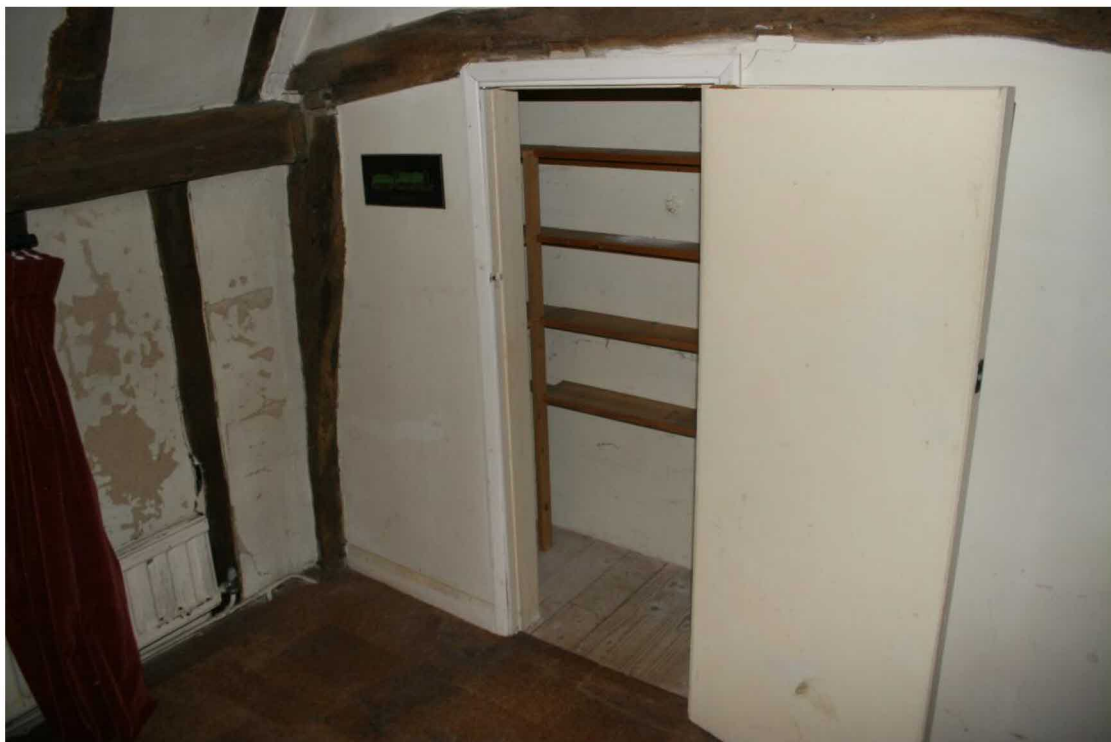
1960's closet. Note the Thistle pink plaster on the wall.
