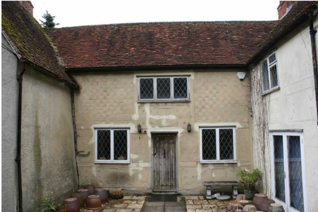
The east elevation of the Hallway Entrance.
