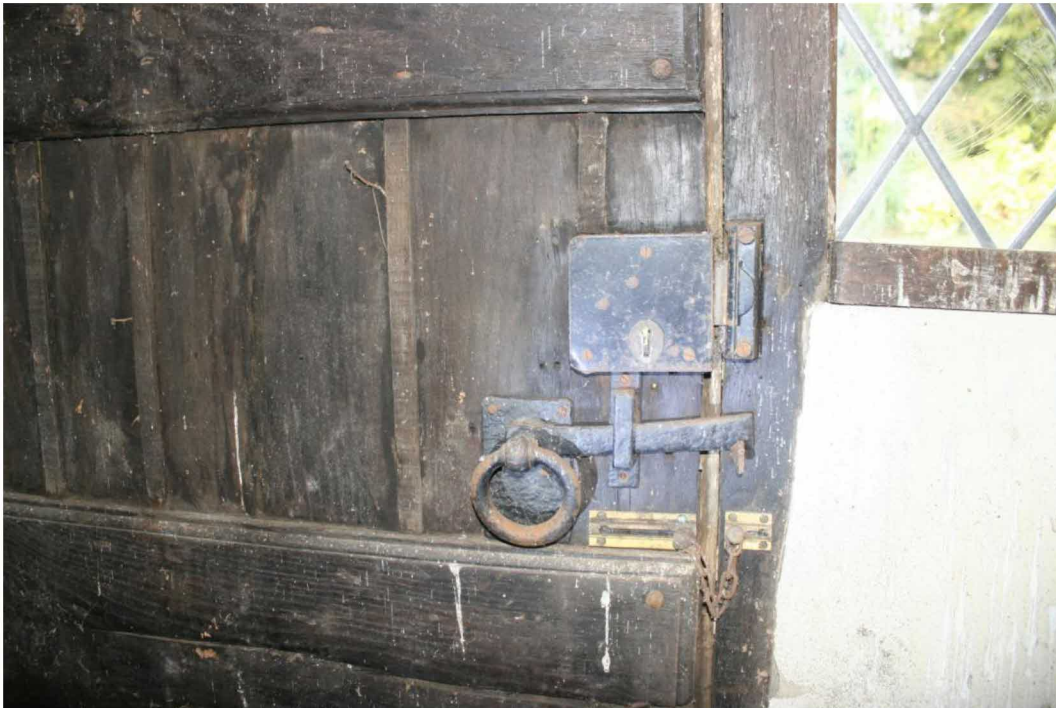
Detail of the inside of the front door.
