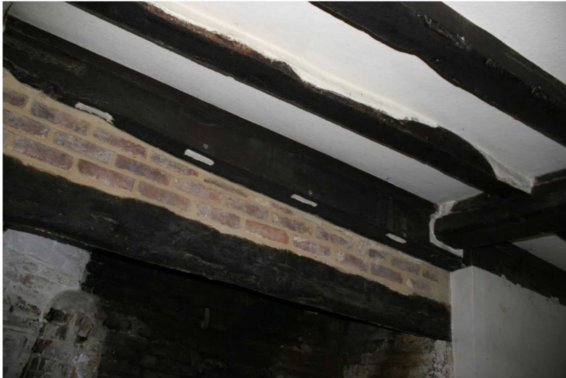
Detail of the framing above the fireplace.
