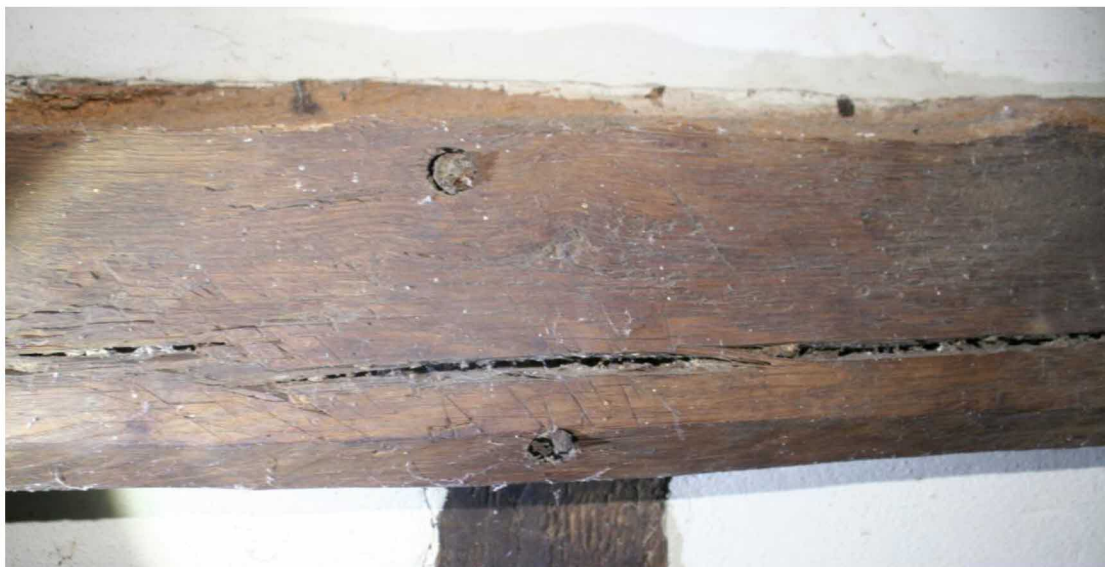
Apotropaic strike marks on the top-plate in the west wall.
