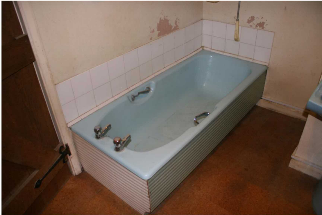
Original 1960's fibreglass bath.
