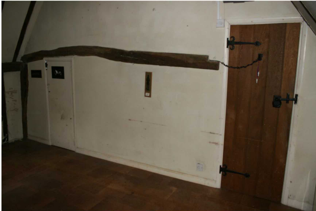
Looking W in the SE Bedroom.
