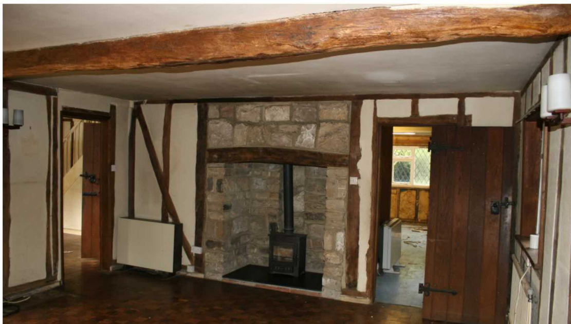
Looking W in the Living Room.
