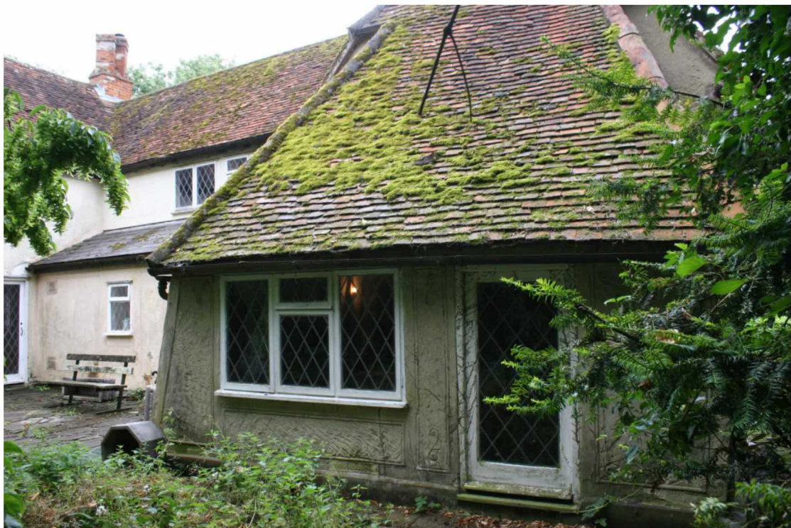
The western elevation of the outshot.
