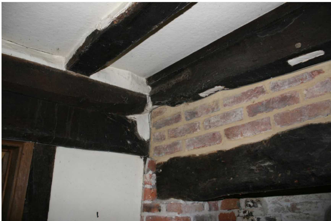
Wrought iron reinforcement on the main joist above the fireplace.
