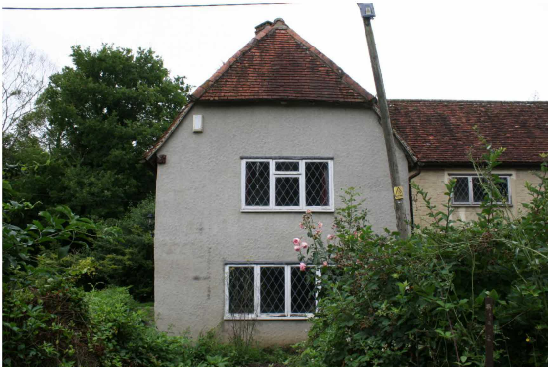
The east elevation of the original cottage.
