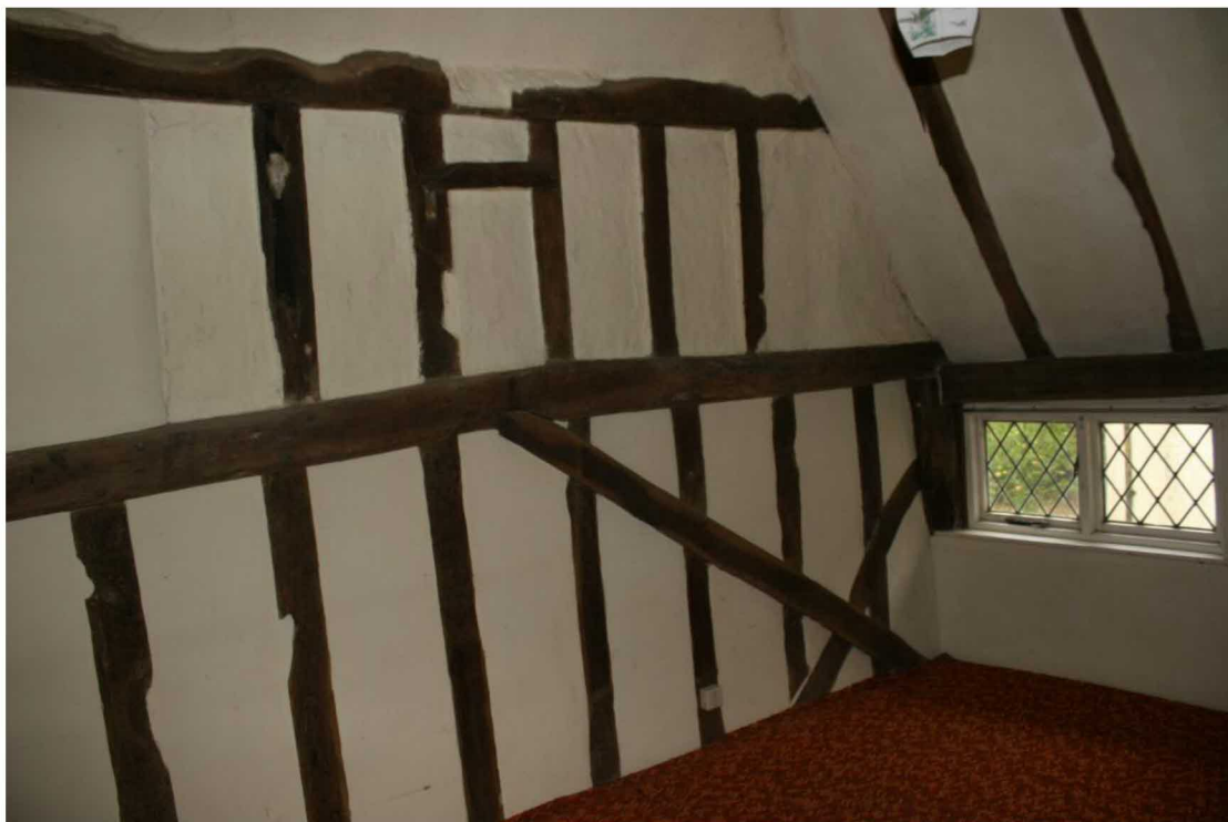
Looking NW in the SW Bedroom.
