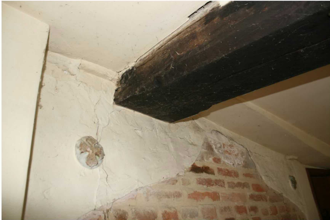
Detail of the main joist with chamfer and notched cyma stops.
