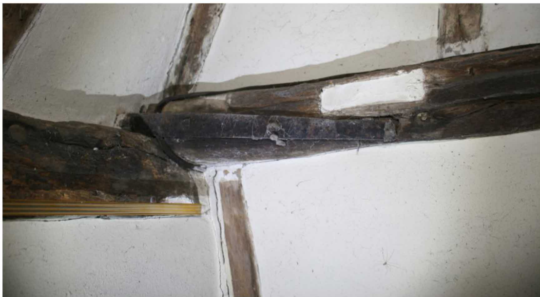
C.19800 wrought iron L-tie in the SW corner of the outshot.
