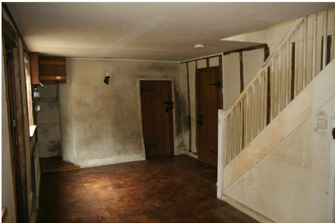
Looking S in the Hallway.
