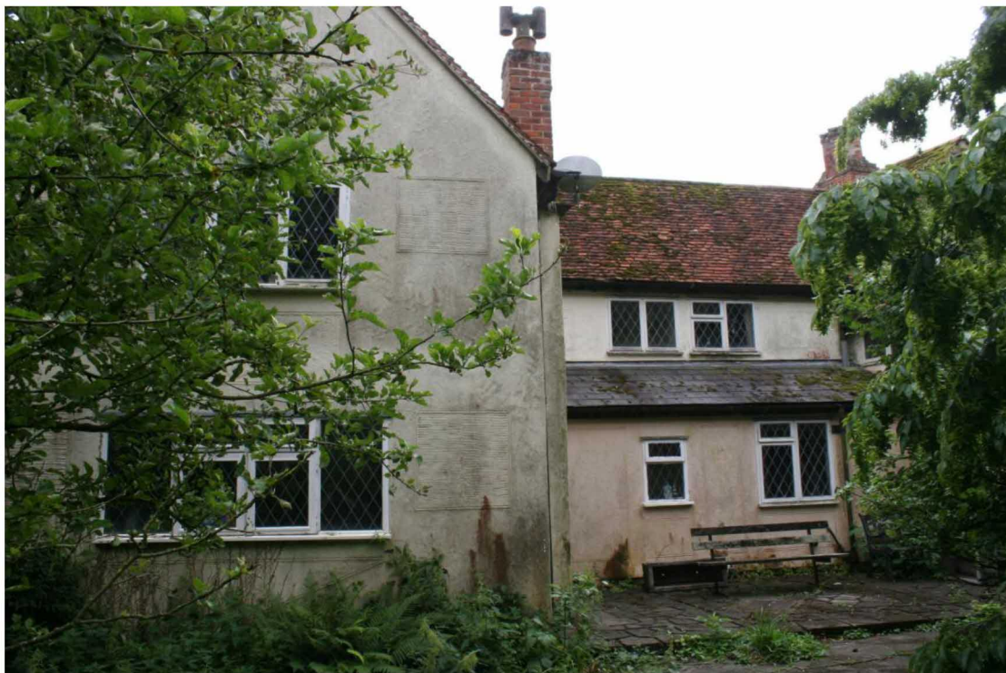
The western elevation of the north range of the 1964 extension.
