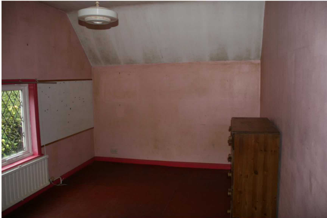
Looking N in the NW Bedroom.
