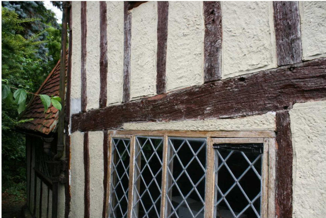
Detail of the midrail and the oak framed windows.
