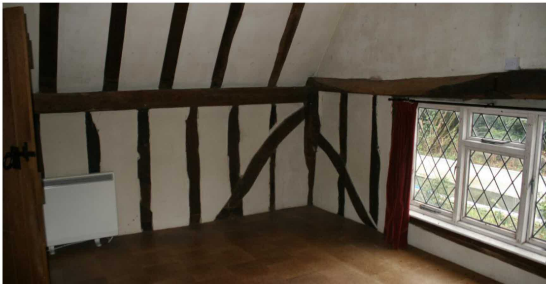
Looking NE in the SE Bedroom.
