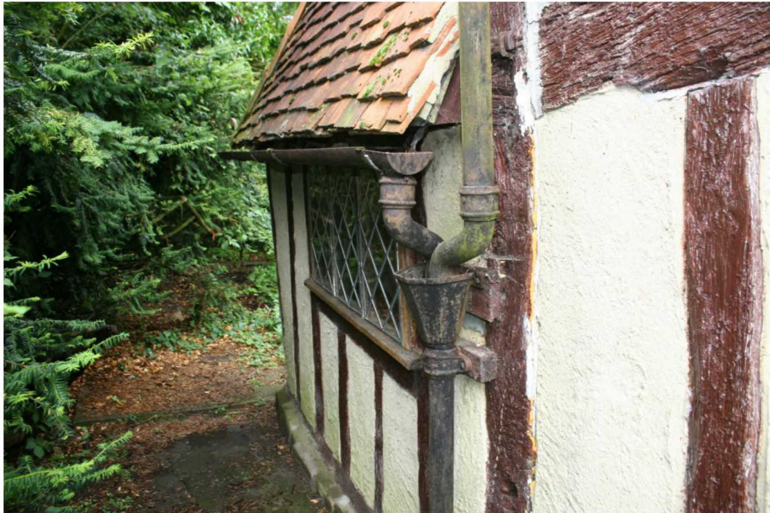
The south elevation of the western outshot.
