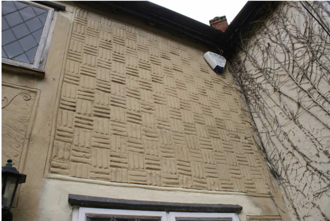
Block printed chequer-work on the east elevation.
