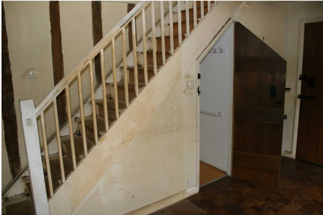
The downstairs bathroom is accessed under the 1964 staircase.
