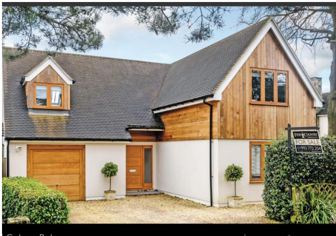
Photo 4 -6 Cadogan Park completed with 2 storey gable
