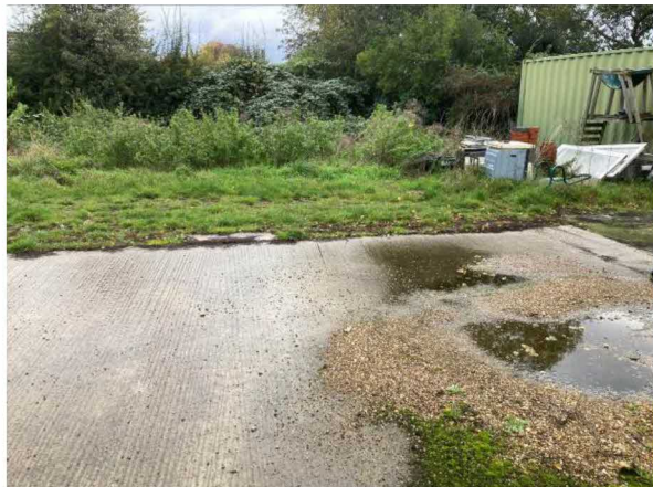
Concrete pad at eastern end of site
