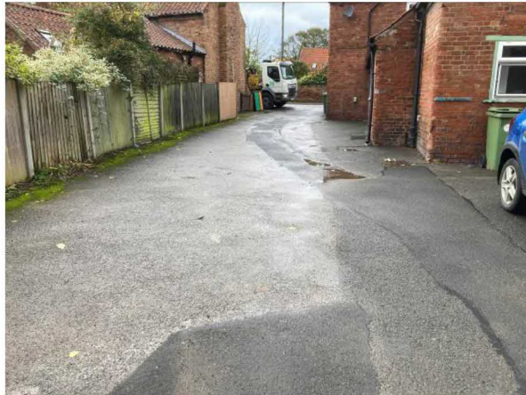
Access from High Street
