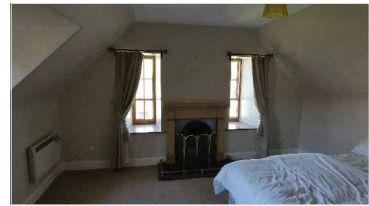
Internal View of Venetian Window
