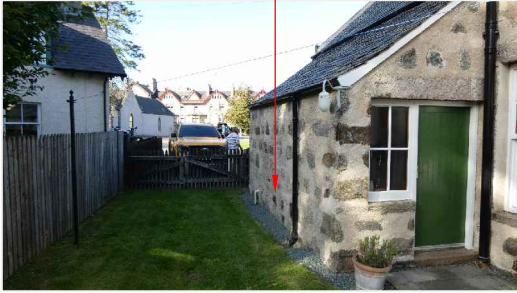
West Elevation of Utility Room Wall
