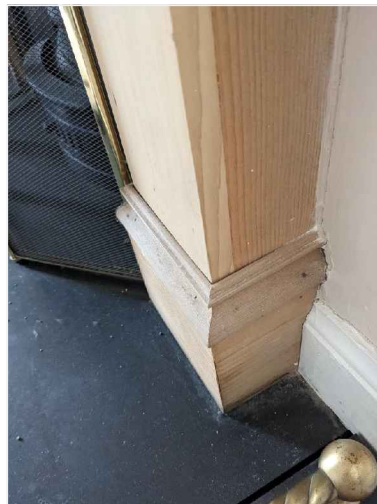
New base block to Fireplace Surround
