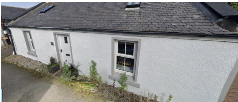
11 South Street, White Render Walls, uPVC White Windows and Black uPVC Rainwater Goods
