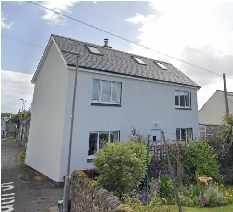
16 South Street, White Walls, White uPVC Windows, Black uPVC Rainwater Goods - Note also the rooflights.
