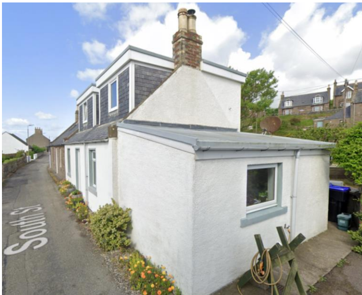
17 South Street, Flat Roof, White Walls, uPVC White Windows and uPVC rainwater Goods
