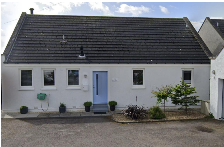
27 South Street, White Walls, White uPVC Windows and Black uPVC Rainwater Goods
