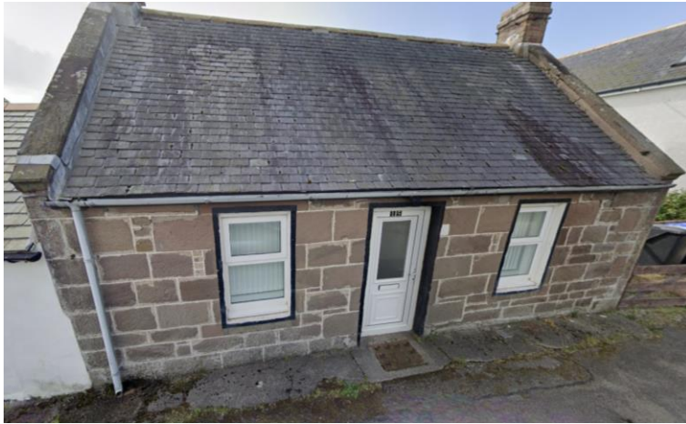
15 South Street, white uPVC windows and uPVC rainwater goods
