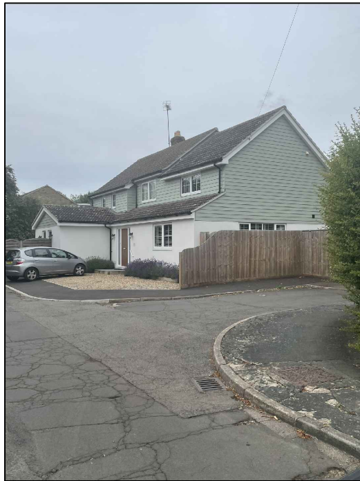
No.16 - Two storey gable extension and single storey front extensions together with full cladding in green horizontal boarding. SIGNIFICANT MASS AND VISUAL IMPACT ON STREET SCENE
