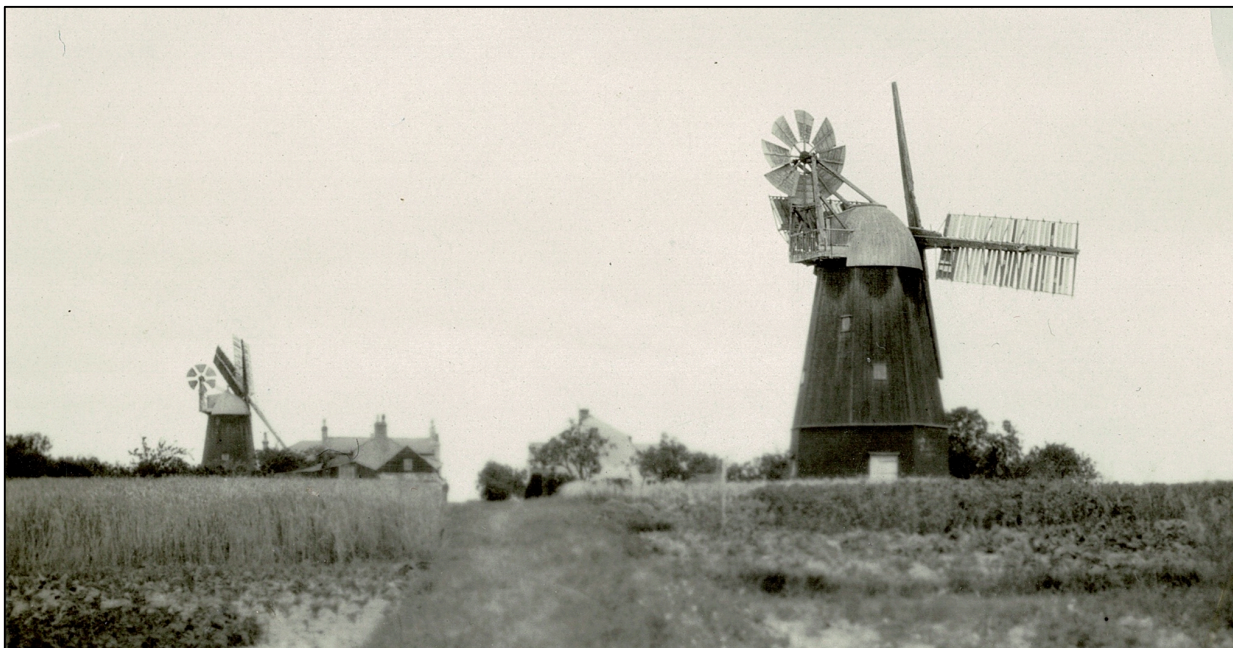
Figure 1: Swaffham Prior windmills c1925, photographed looking up the track towards the north west. The tower mill is on the left and the smock is on the right. The smock has lost one pair of sails but is otherwise in working order and the fantails of both mills are working correctly as they are both facing the same direction. (Mills Archive Rex Wailes Collection)
