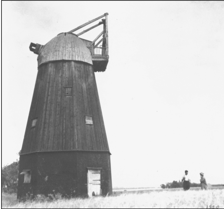
Figure 3: Swaffham Prior smock mill following the removal of the sails, photographed by Harry Meyer in 1935 (Mills Archive).
