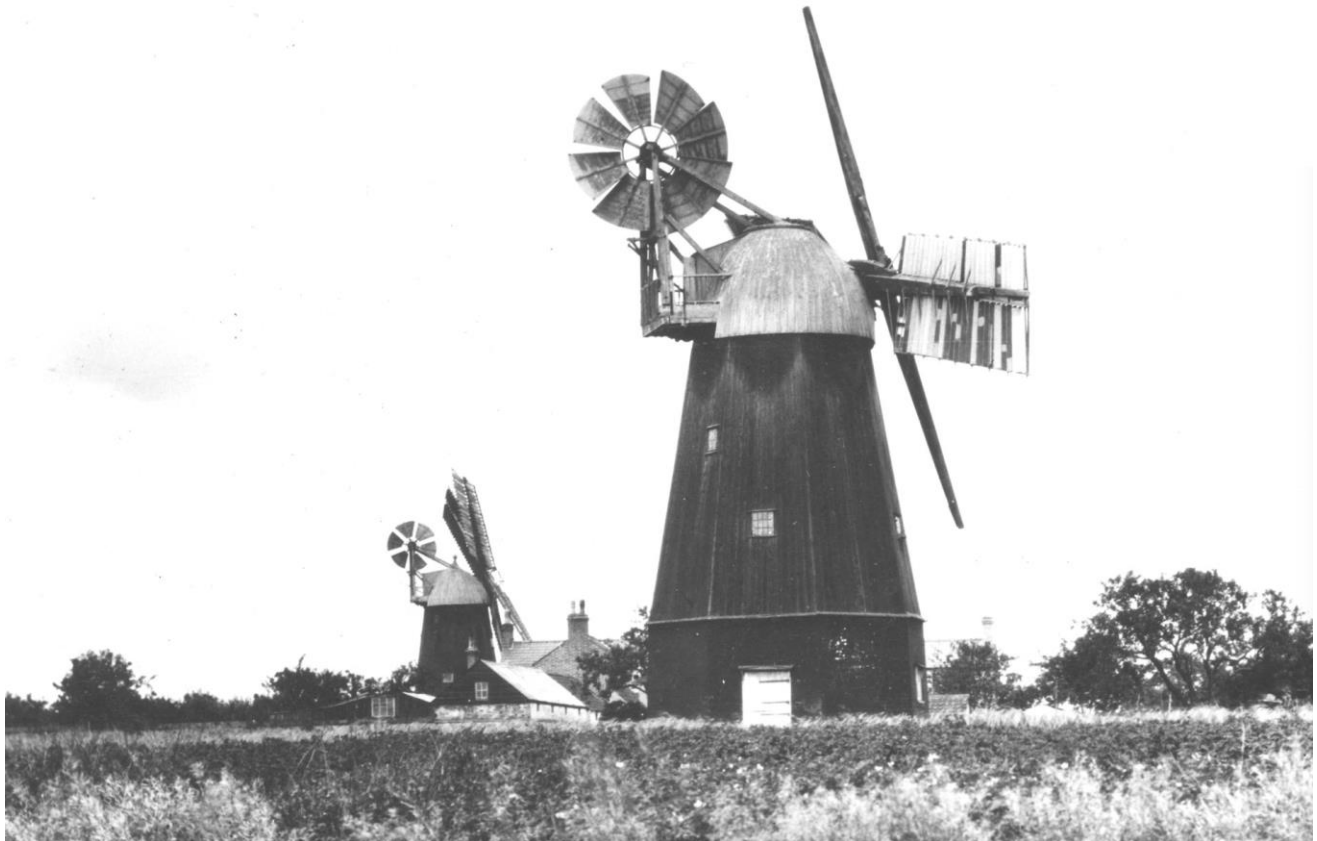
Figure 1: Swaffham Prior windmills circa 1920. Foster's tower mill is in the background. The smock mill is in the foreground. It has reached the end of its working life and has already lost two of its sails.
