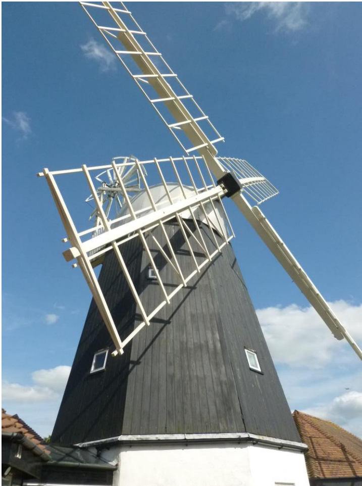
Figure 2: The smock mill as converted, showing its non-working 'dummy' sails (October 2019).
