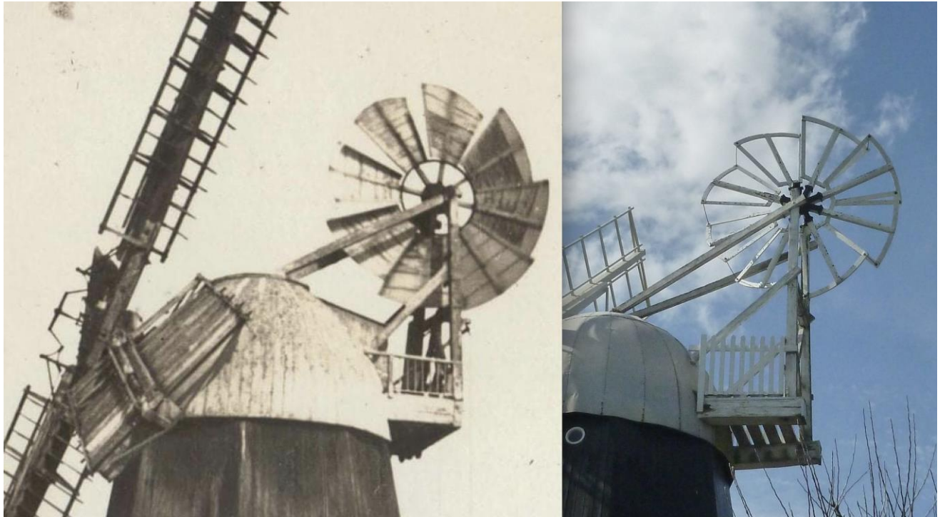
Figures 3a and 3b: The original (left) and present cap roof and fantail compared.
