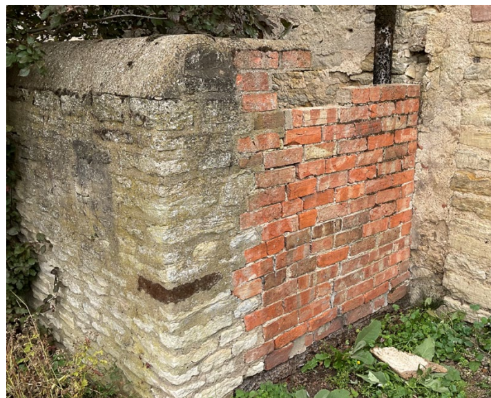
Plate 12: Section of infill brick wall to be removed.
