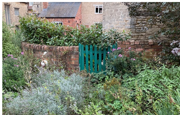
Plate 13: Section of wall to be infilled.
