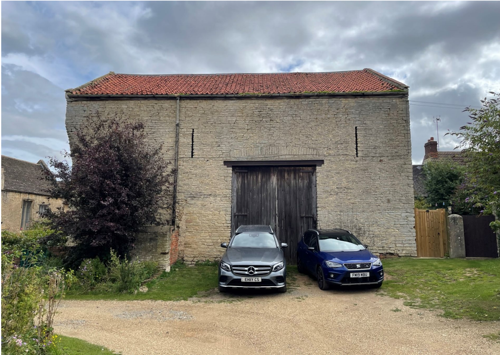
Plate 6: Barn, west elevation.
