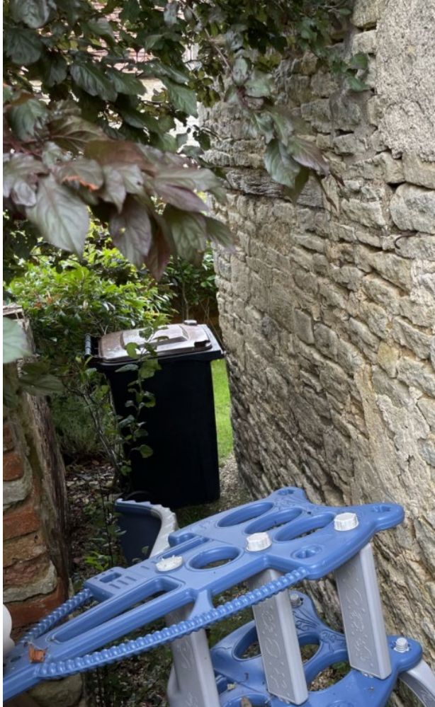
Plate 10: Previously blocked opening to be reopened and lintel raised.
