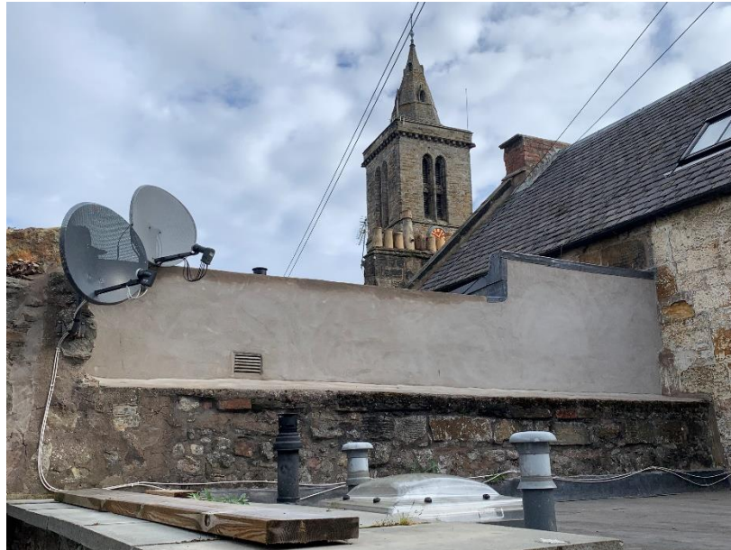
Boundary Wall, after works carried out
