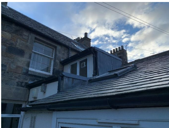
Rear extension roof, 2022
