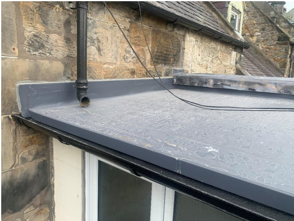
New single ply roof installed July 2023
