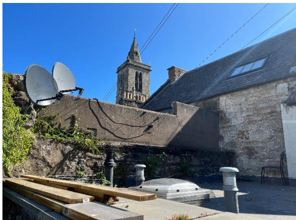
Boundary wall before works, June 2023
