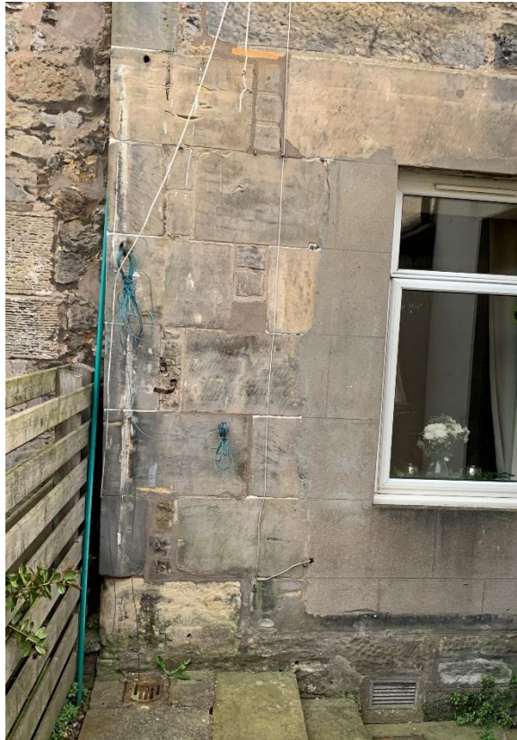
Former location of RWP, ties still left on wall
