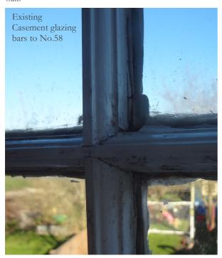
Purpose made timber joinery, predominantly with slim glazing bars and pentice boards cappings, with the dormer and ground floor lean-to window of a mullion design.
