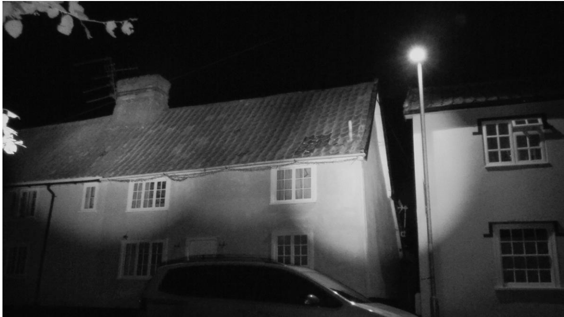
Photo 1 , screenshot from infrared camera on the west aspect. 24 th August 2023.
