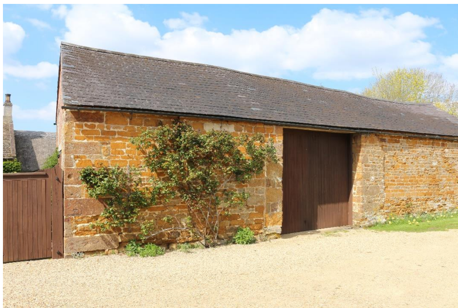
Figure 21: Southern elevation of barn
