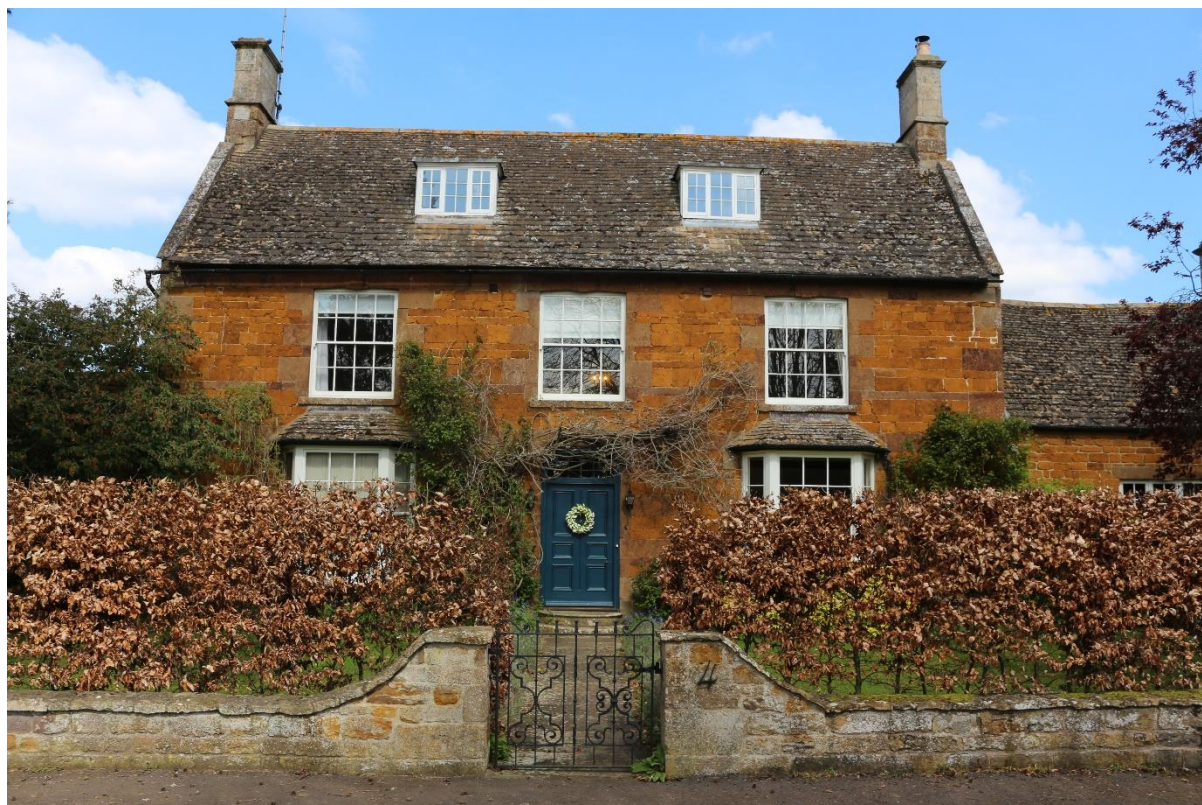
Figure 13: Principal elevation of the Bell House
