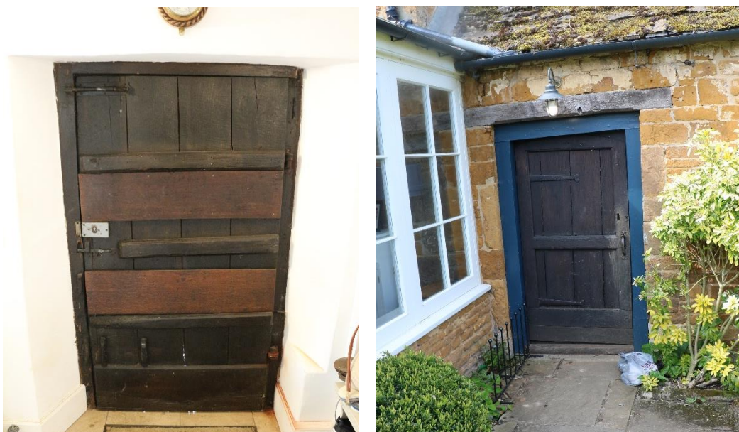
Figure 28: Internal and external view of door in G.11
