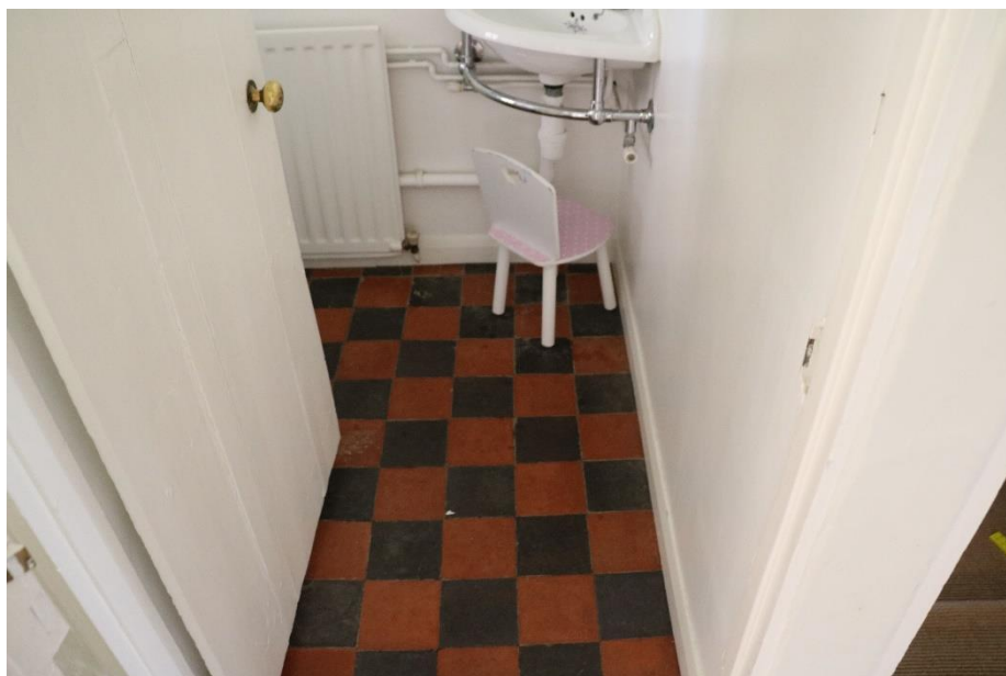
Figure 36: 19th century quarry tiles in downstairs toilet
