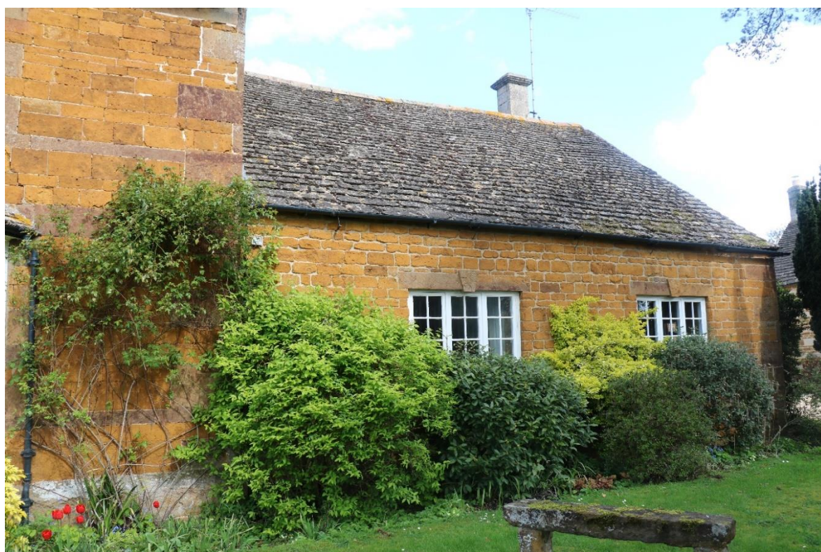
Figure 14: Southern extension to frontage of main house
