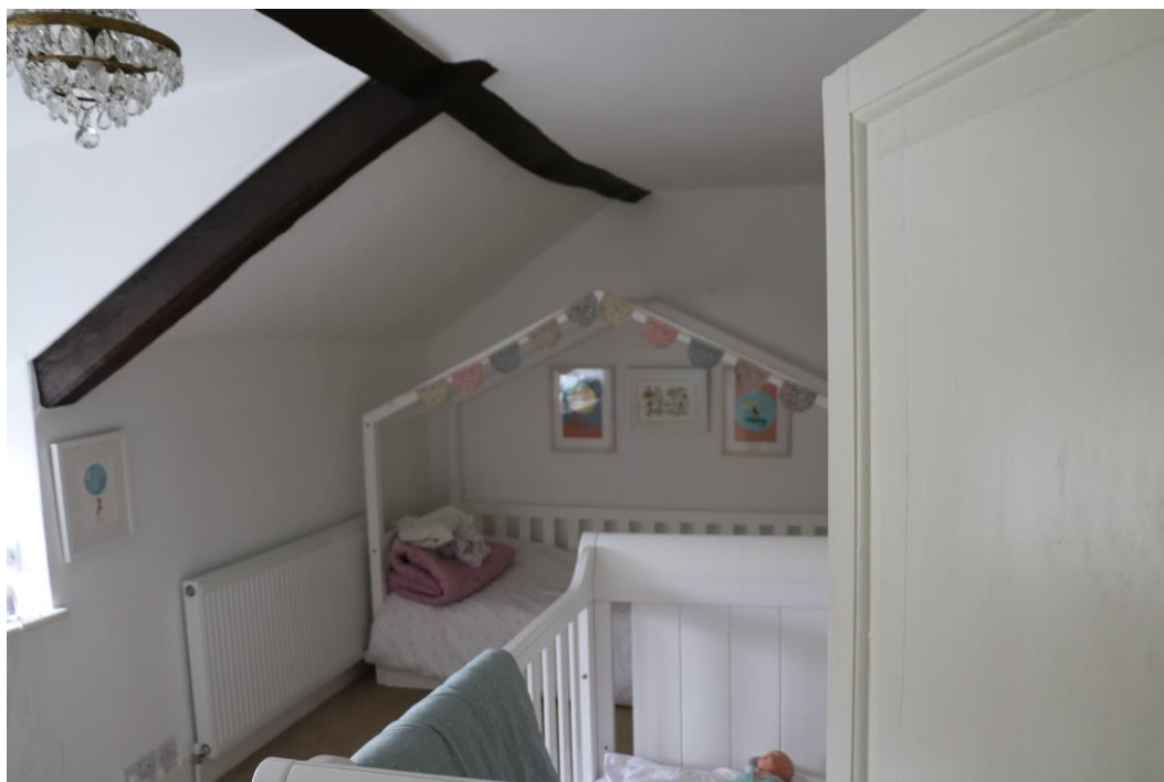
Figure 38: Historic beams to room 1.4
