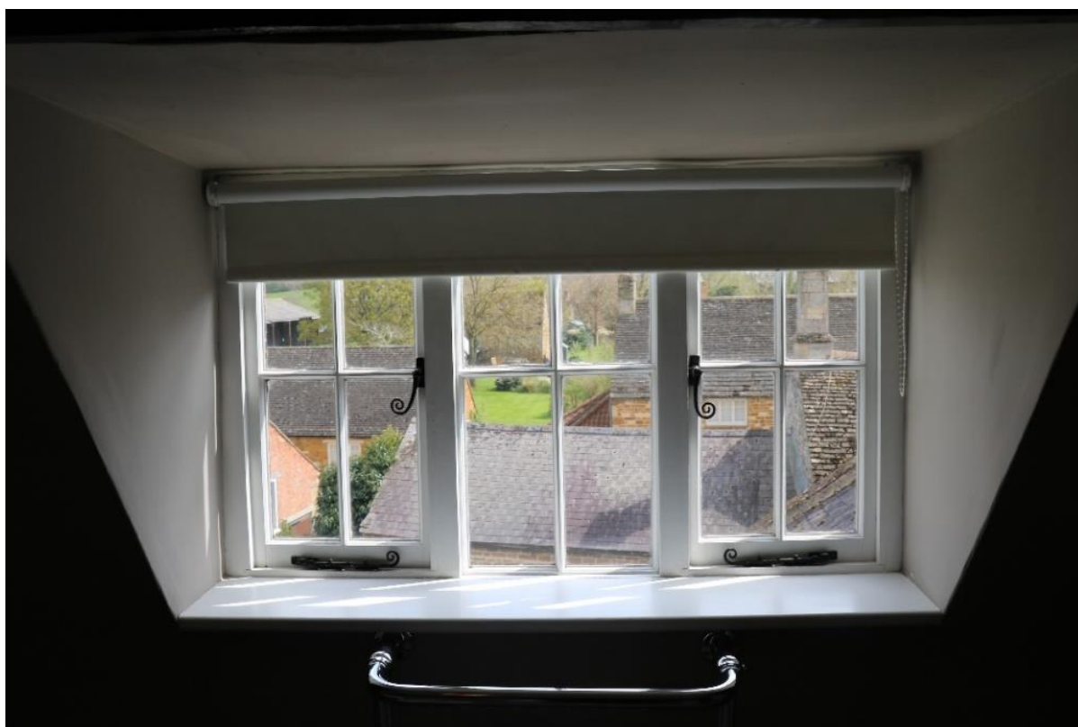
Figure 29: 20th century dormer to second floor at rear
