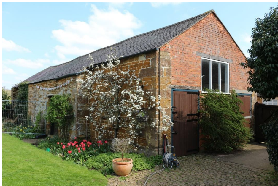
Figure 20: Northern elevation of barn
