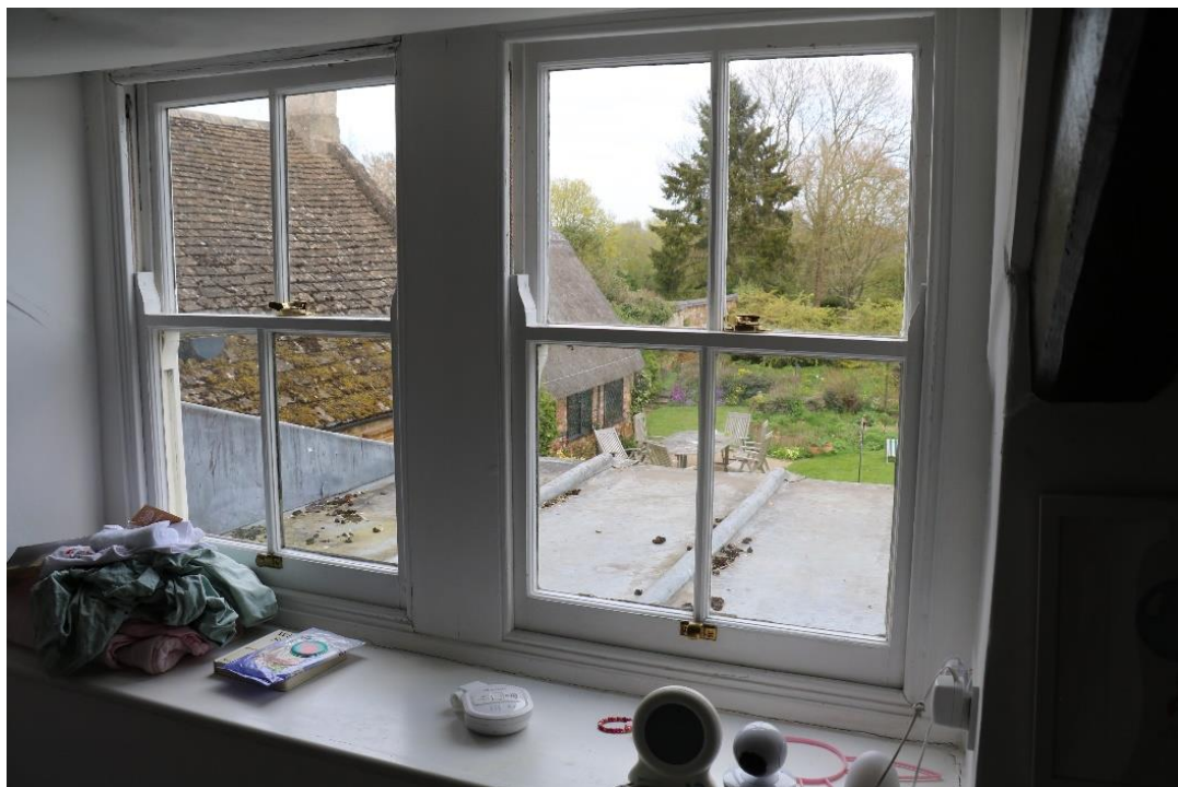
Figure 31: Window to room 1.4
