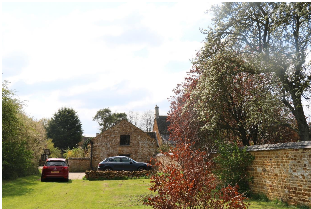
Figure 52: View south-west from the scheduled monument towards the rear of the Bell House
