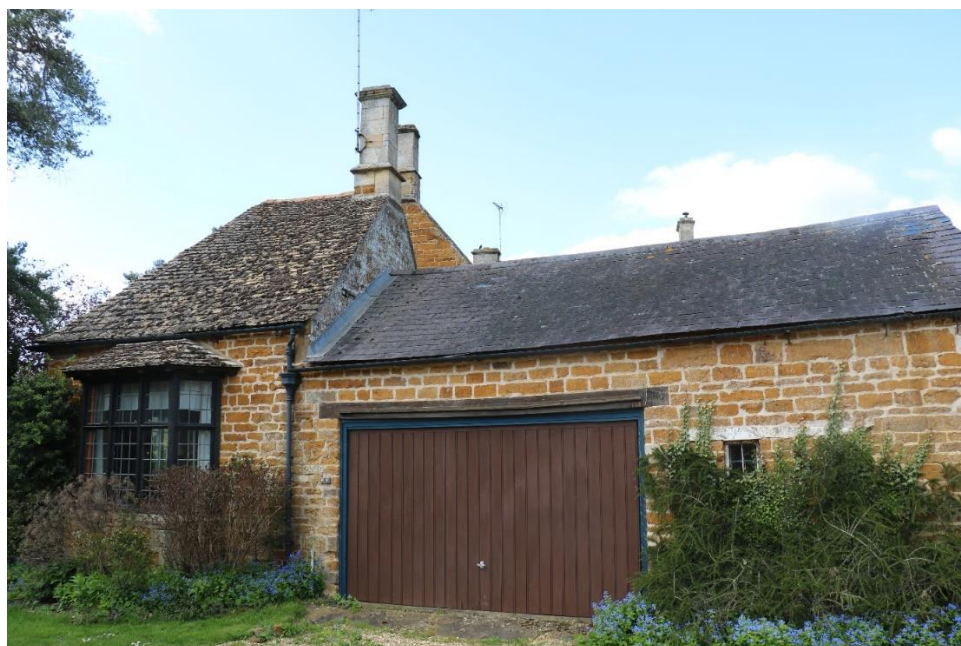
Figure 19: Southern elevation of extension and garage
