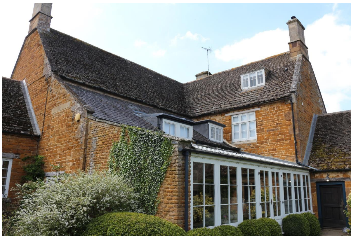
Figure 16: Rear elevation of main section of house
