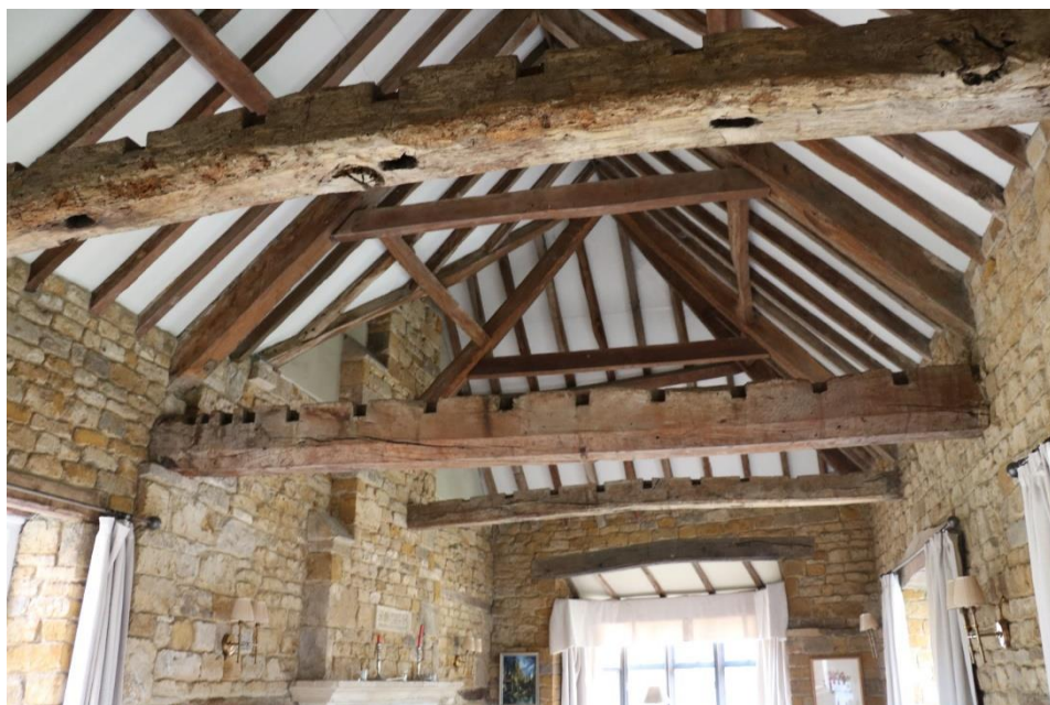
Figure 37: Exposed roof structure in G.2
