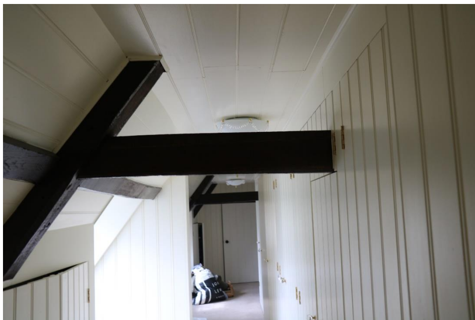
Figure 40: Historic beams to room 2.1
