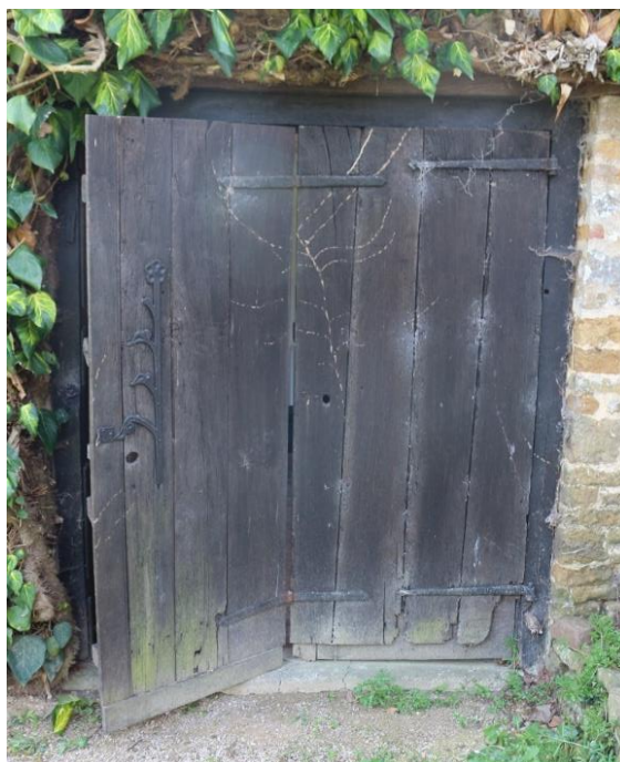
Figure 25: Door to room G.13
