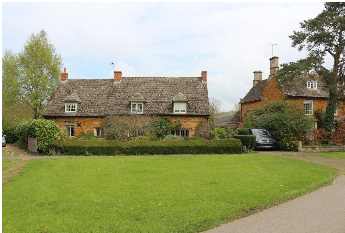
Figure 49: Principal elevation of Lincoln House
