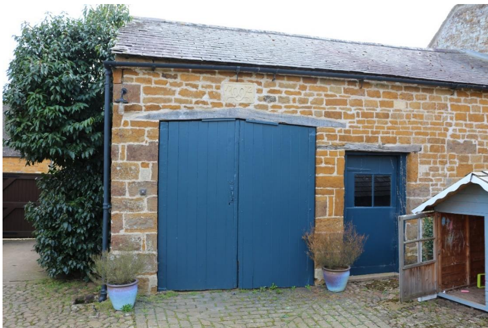
Figure 18: Northern elevation of garage
