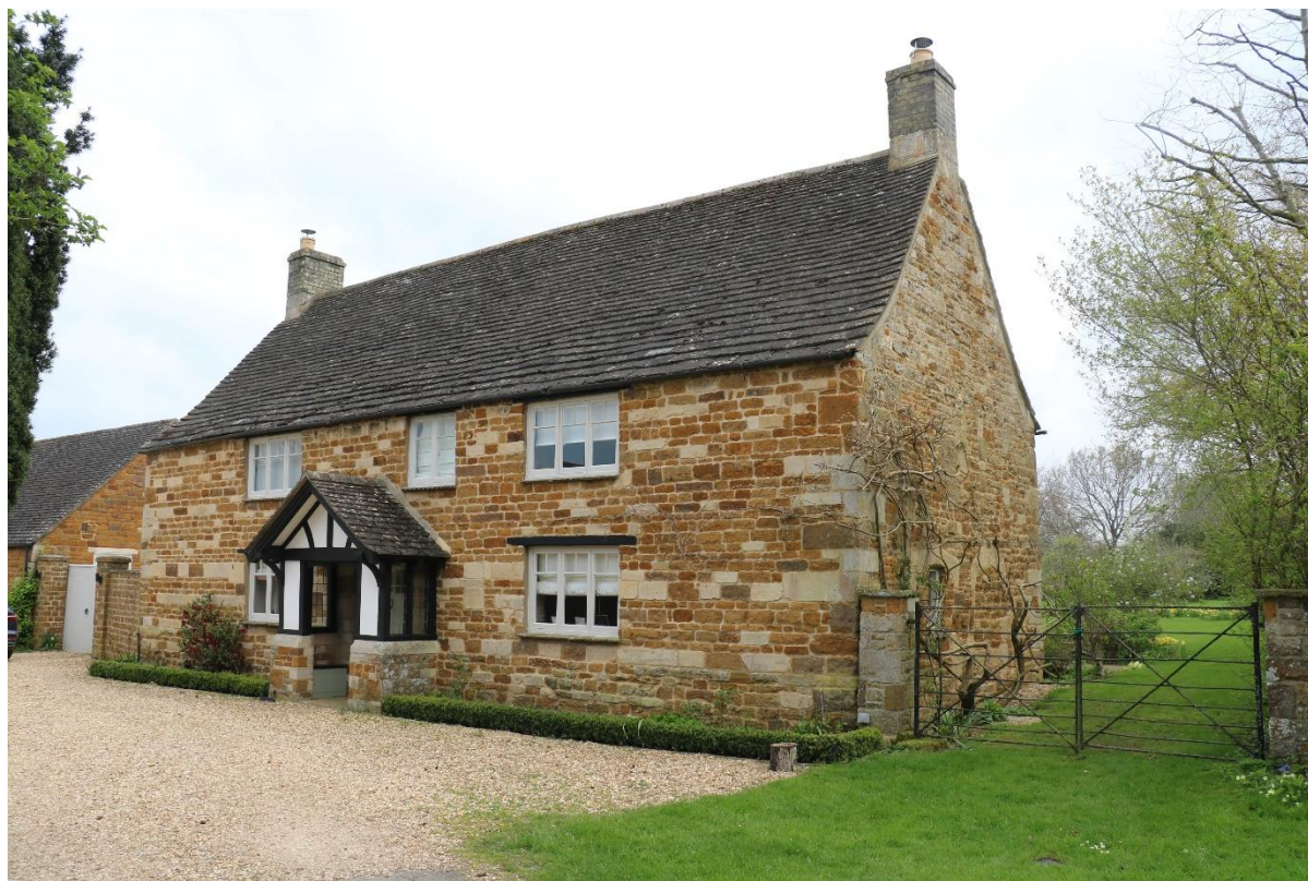
Figure 46: Principal elevation of Stoneleigh
