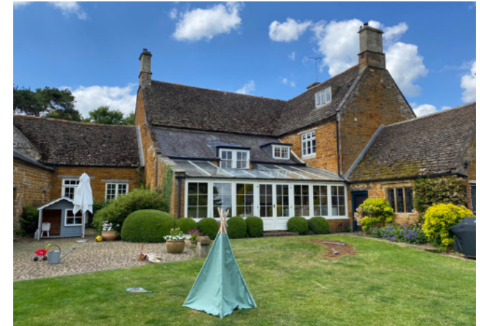
View of the Existing Rear Elevation showing the interrupted heritage with the modern extension.
