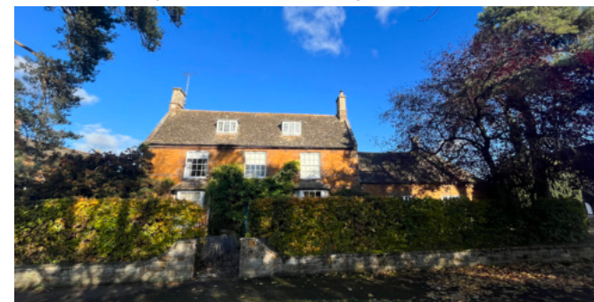
Existing Street View of the Application Site
