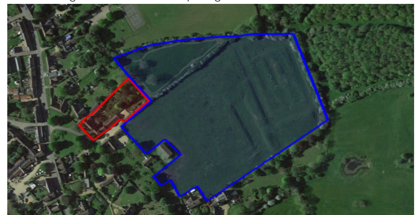
Google Earth Ariel View of the Site in Red and Land Owned by the Client in Blue
