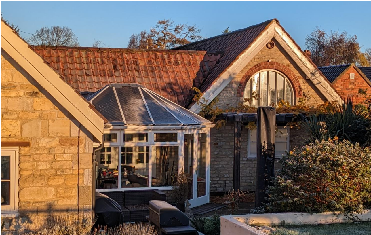
Photograph showing existing conservatory that is proposed to be replaced.
