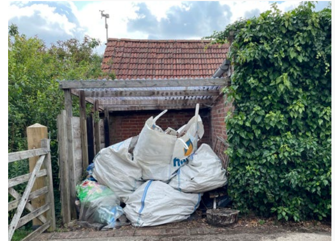
Canopy attached to Wynne Cottage to be removed.
