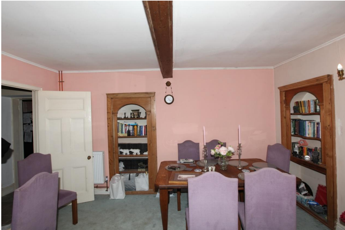
Illus. 17. The rear wall of the dining room showing the arched shelves of stripped pine that were probably installed by the previous owner. The timber is a mixture of old and new, and contains anomalies such as fittings for door hinges. The left-hand unit penetrates the brick wall and may have formed a doorway previously.
