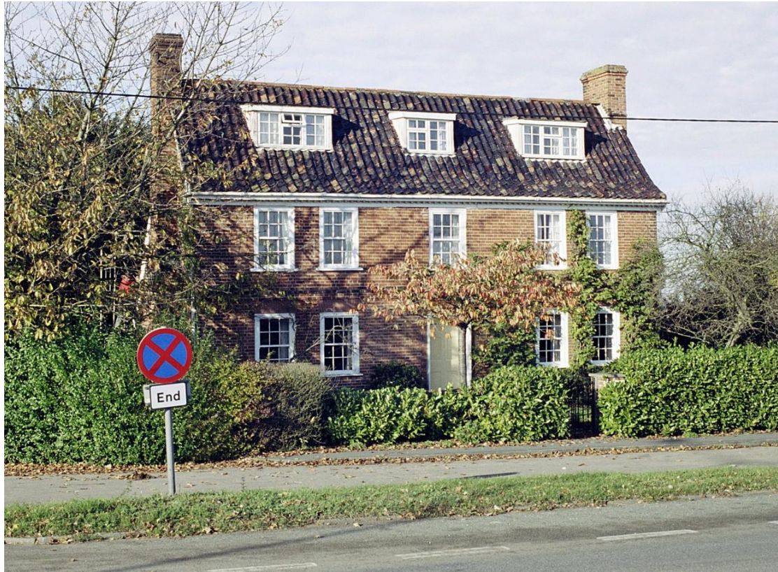
Figure 11. The facade in 2004, looking much as today with separate sash windows to the left and three enlarged dormer windows.
