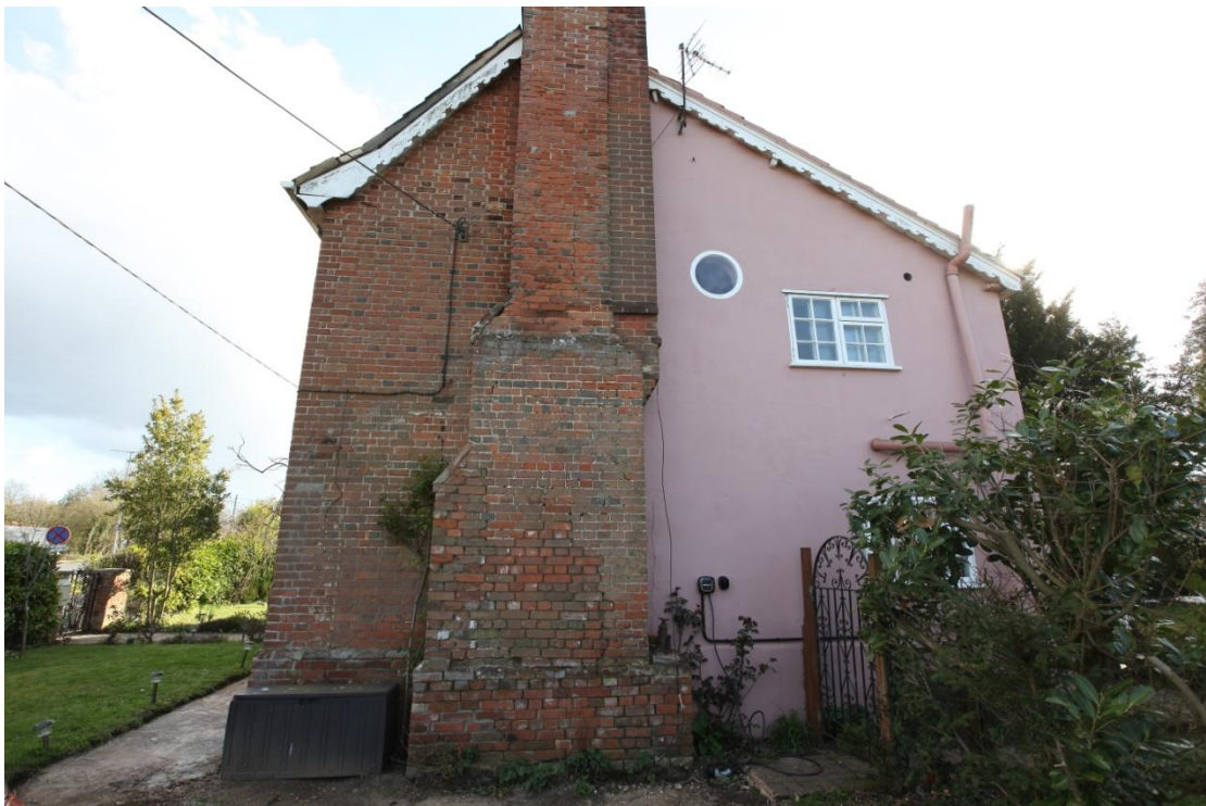
Illus. 8. The northern gable, partly encased in the cement render of the late-20 th century two-storied rear extension. The chimney was previously adjoined by a boarded lean-to shed that may have contained a bread oven (figure 10), and the brickwork of the chimney itself has been much altered. The curious double shaft relates either to the missing oven or an inserted first-floor fireplace of which there is no internal evidence.
