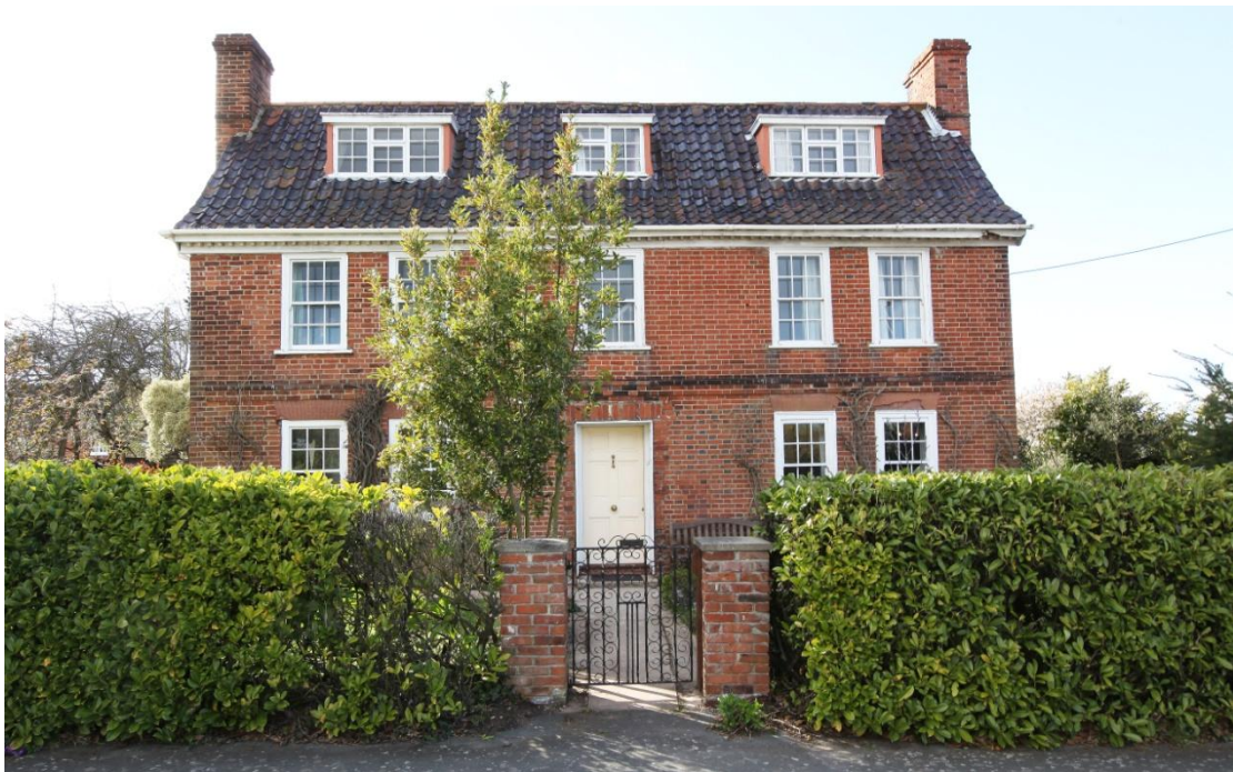
Illus. 2. The eastern facade from the remaining section of the original road between London and Ipswich. The current symmetrical appearance dates only from the mid-20 th century when the adjoining sash windows to the left of the central entrance were separated to match those on the right. In their current form the three dormer windows are also 20 th century additions that replaced the smaller pair in figures 8-10.
