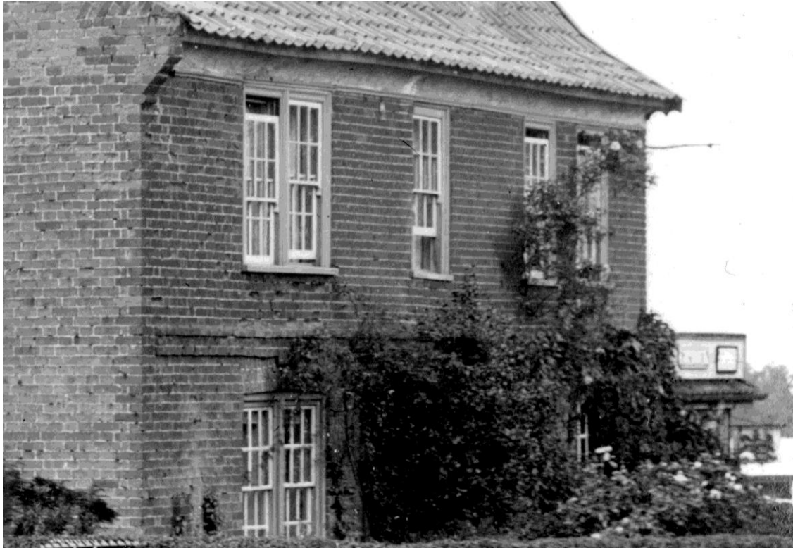
Figure 8b. A detail of the facade in figure 8a highlighting the adjoining sash windows to the left with no evidence of disturbance in the brickwork on each side. The first-floor upper sashes were provided with horns in the manner of the mid-19 th century and later, although they are absent from those on the ground floor. What appears to be a single-storied shop with signs above its awning is visible to the right.
