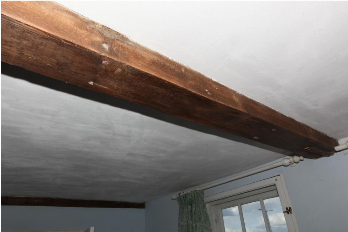
Illus. 23. A detail of the pine binding joist of bedroom 1, which contains vertical pegs and scored lines for the concealed common joists above. The unusually plain nature of this timber suggests it was concealed by moulded planks like those which survive elsewhere in the house.
