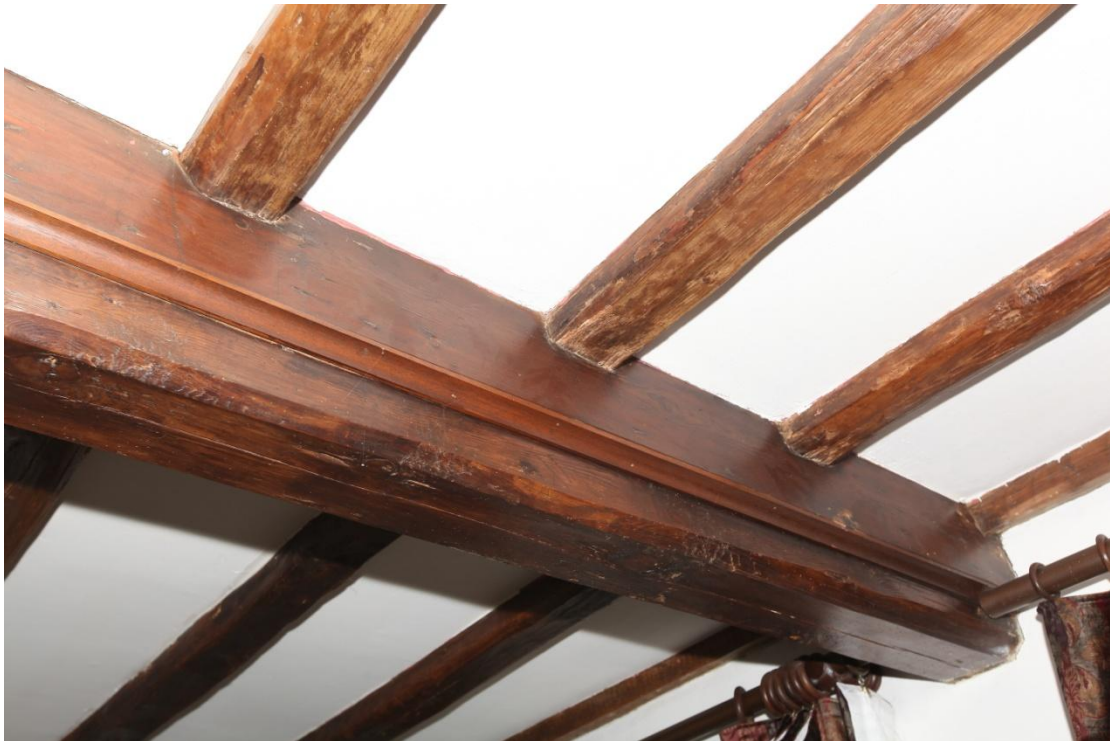
Illus. 16. A detail of the neatly chamfered binding joist between the windows of the sitting room in illustration 15 with later boards concealing the joints of the common joists above. The pine timber appears authentic and may have been boxed at some point. The roughly hewn pine common joists are also convincing, and match the rafters in illustration 26, but there is no evidence of the plaster that might have been expected in a house of this period and quality.
