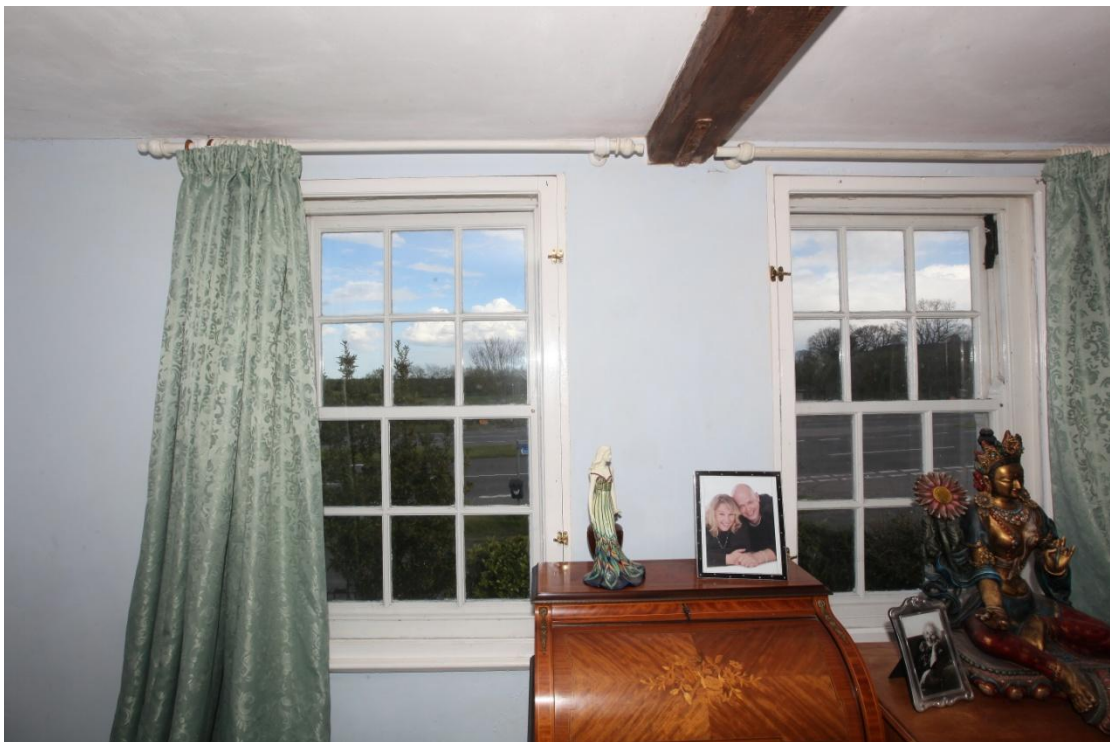
Illus. 22. The 20 th century windows in the front wall of bedroom 1. As in the sitting room beneath, there is no obvious evidence of the partition that might have been expected given the crowded nature of the blacksmith's cottage in the 19 th century.
