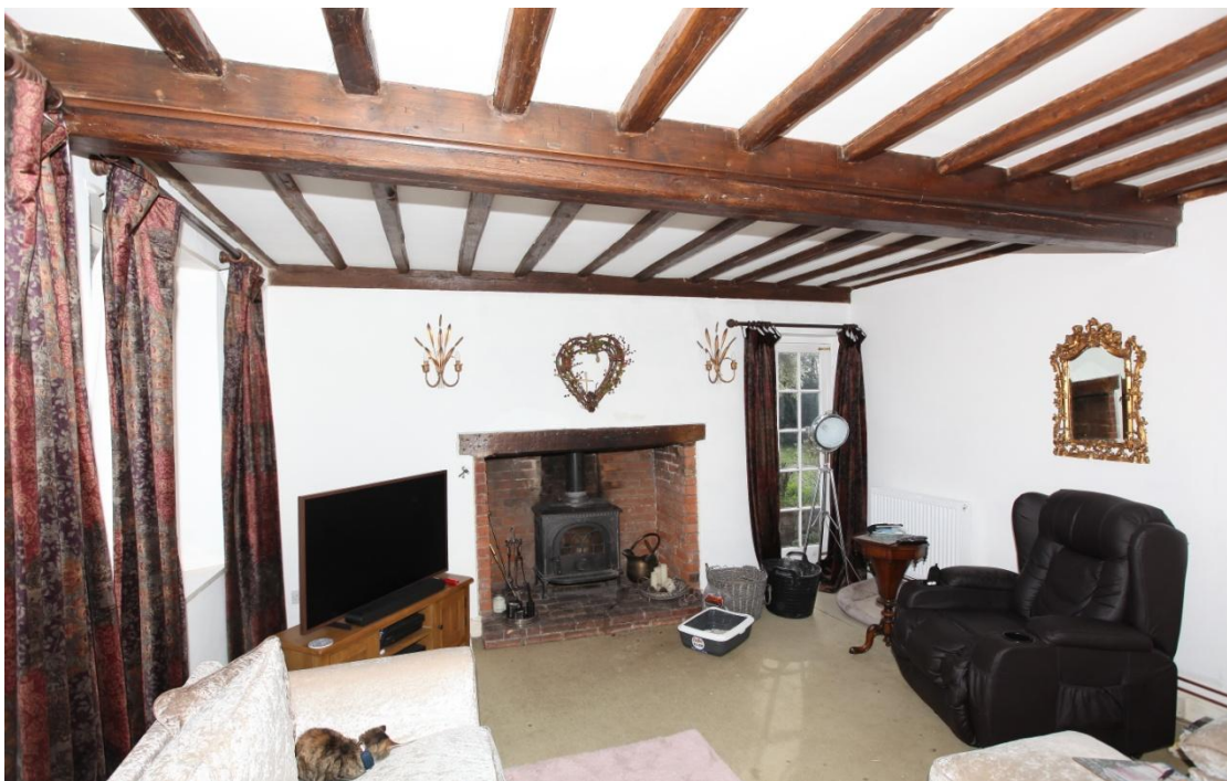
Illus. 14. The sitting room's southern gable showing the modern glazed door in the entrance to the blacksmith's cottage. The brickwork of the fireplace is consistent with the early-19 th century but the lamb's tongue chamfer stops of its lintel are more typical of the 17 th century and it may have been imported – although it fits the brickwork.
