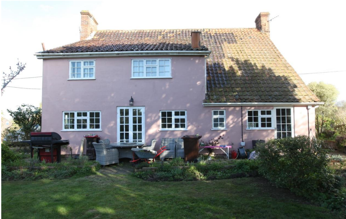
Illus. 11. The house from its rear garden with the late-20 th century two-storied extension on the left. This consists of cement blocks and must date from the 1970s or 80s. The single-storied structure contains matching windows but probably reflects the height of the original rear lean-to on the historic maps. However, it must represent a replacement as both rear corners were indented on the maps (indicating the previous structure shopped short of the gables).
