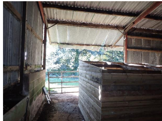
Figure 5. The large opening to the southwest elevation
