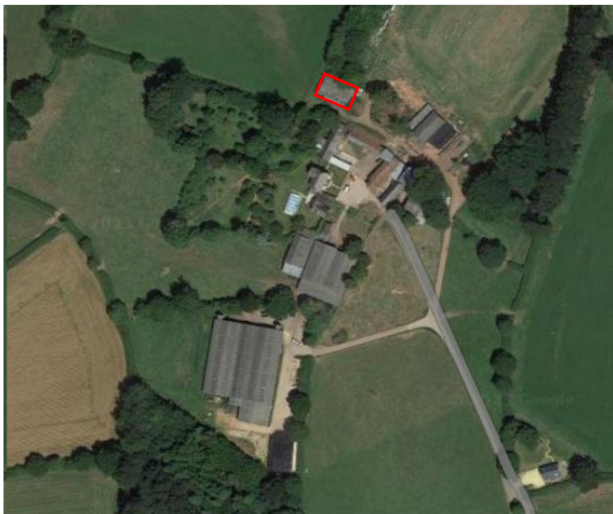
Figure 1. The location of the agricultural barn at Peradon Farm highlighted in red
