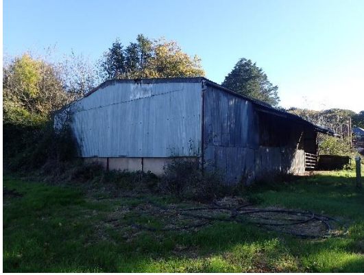
Figure 2. The barn viewed from the west
