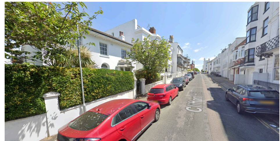
View of Clifton Hill Looking East
