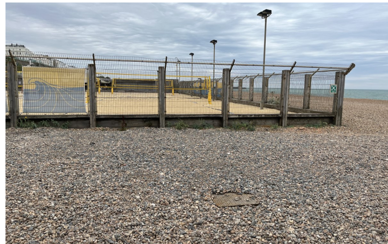
Figure 10: View looking east of adjacent boundary fence
