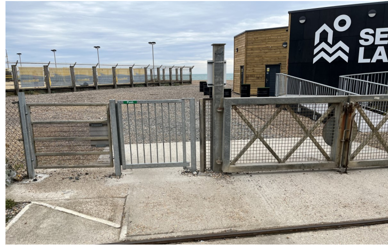
Figure 8: View of pedestrian and vehicle railway crossing gates
