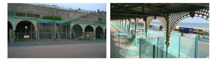
The structure of the terrace is now considered unsafe and has been closed off awaiting significant conservation works. The Madeira Lift was refurbished a few years ago and the shelter building operates a successful bar and music venue.
