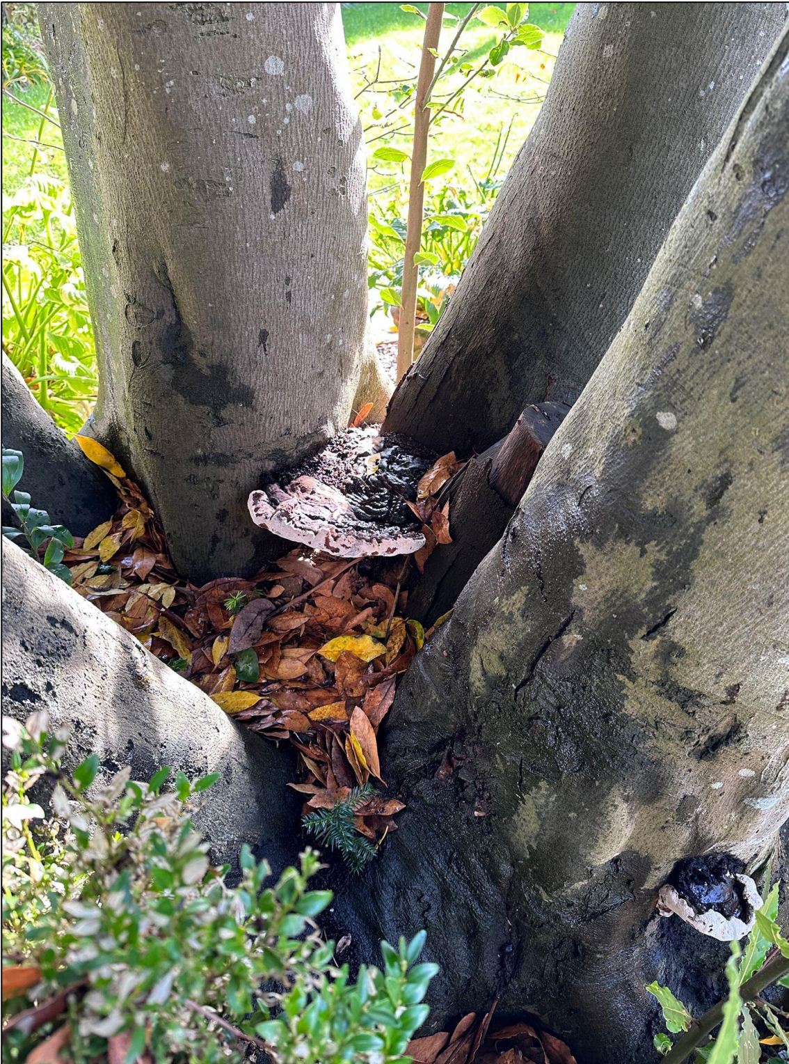
Photo three – Ganoderma spp. to internal base of tree.
