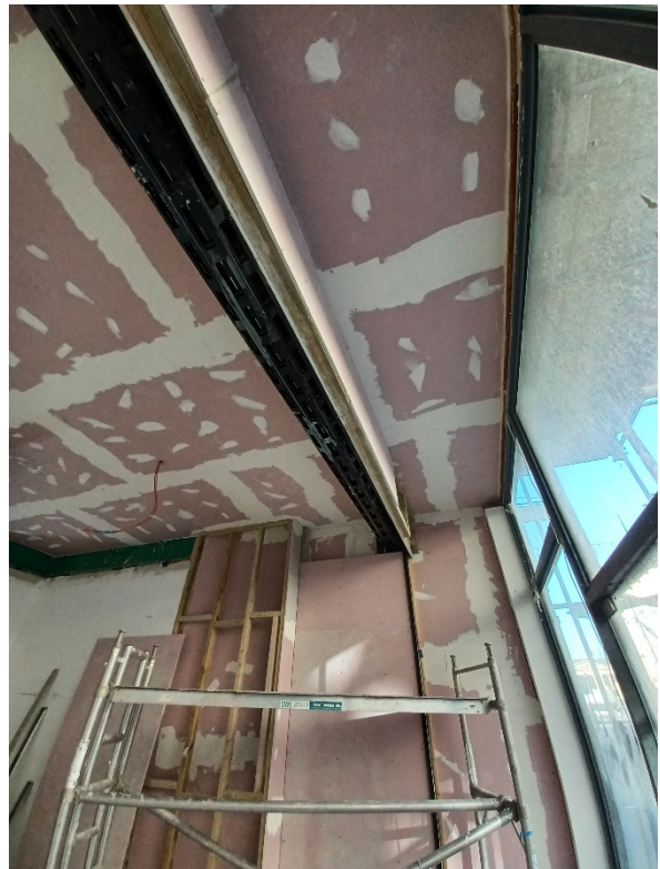
Photograph 17 – Preparatory framing to party wall
