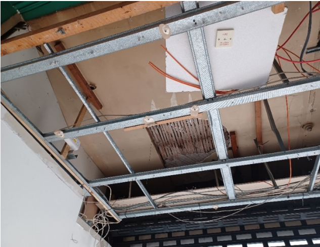
Photograph 5 – General view of exposed soffit
