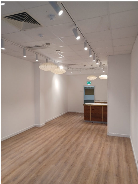
Photograph 20 - General view post reinstatement of suspended ceiling
