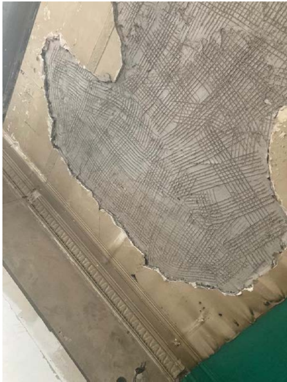
Photograph 10 – First coat plaster repairs
