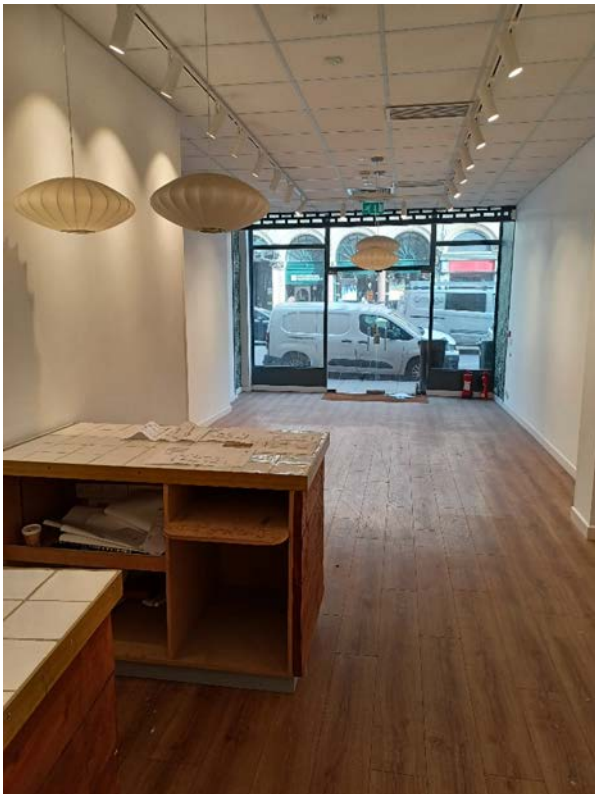
Photograph 1 – Main retail area (Suspended Ceiling)
