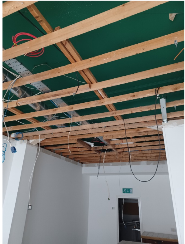
Photograph 8 – General view of sub-frame
