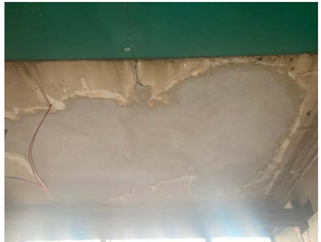
Photograph 13 – Completed plaster repairs
