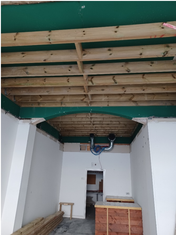
Photograph 14 – General view of new independent sub-frame
