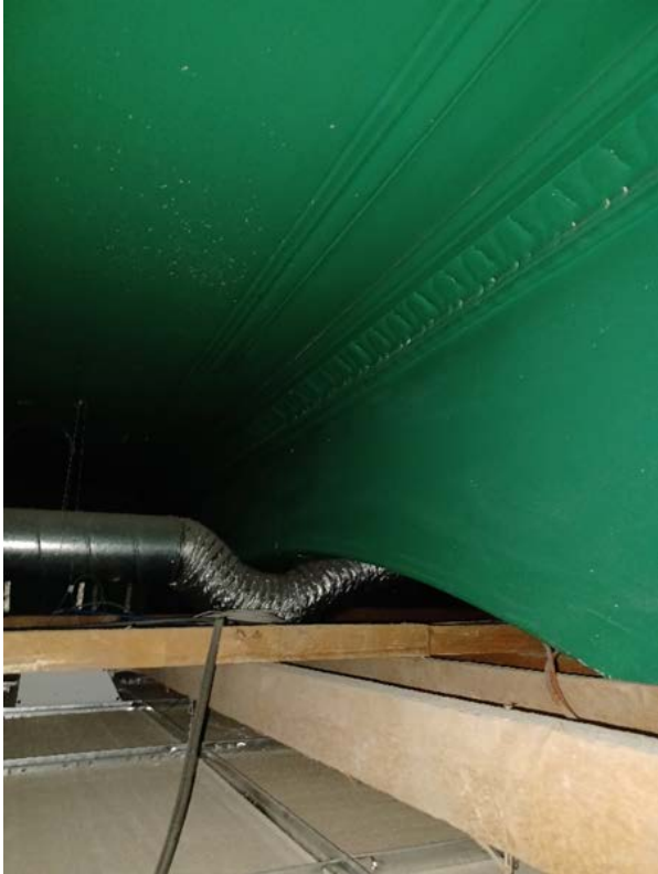
Photograph 3 – Example of lath and plaster ceiling over main retail space
