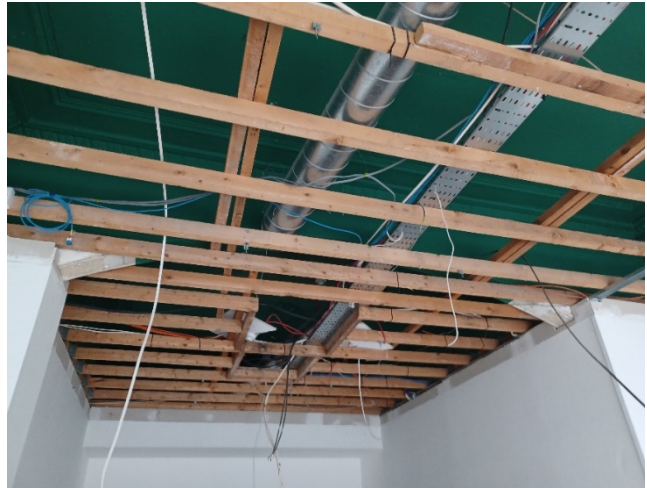
Photograph 6 – Previously installed timber subframe
