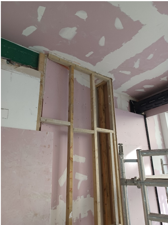
Photograph 16 – Preparatory framing to party wall
