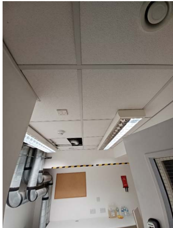
Photograph 2 – Rear Store Area (Suspended Ceiling)
