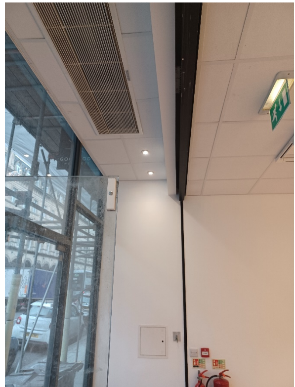
Photograph 19 – Shopfront area post reinstatement of suspended ceiling
