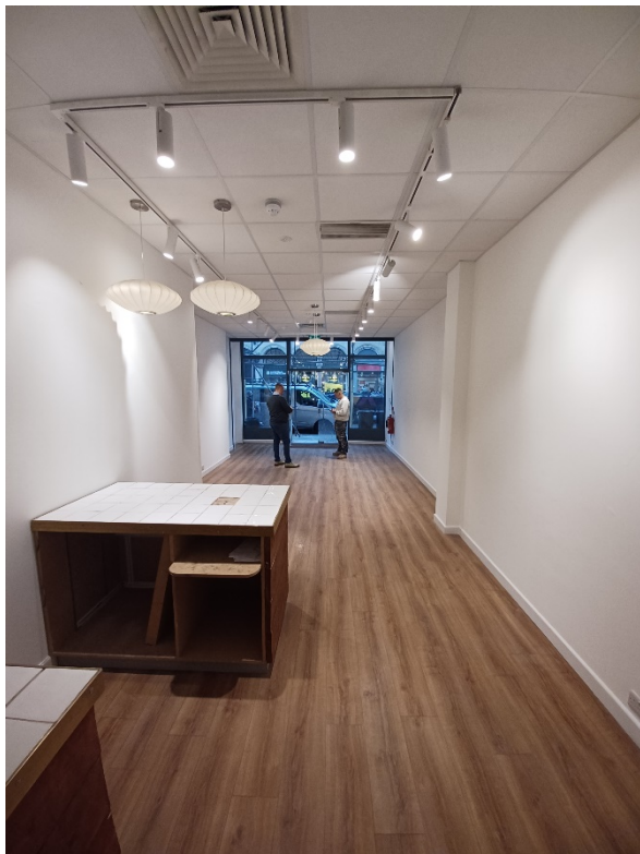
Photograph 18 – General view post reinstatement of suspended ceiling
