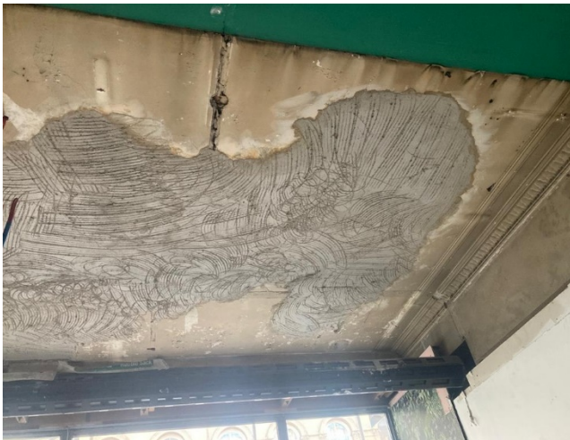
Photograph 12 – Second coat plaster repairs
