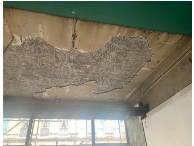
Photograph 11 – First coat plaster repairs
