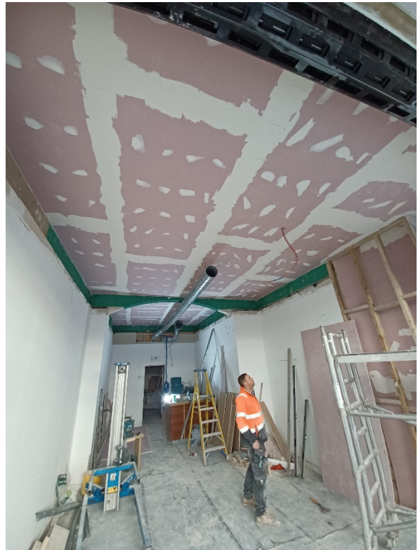
Photograph 15 – Fire board installed to new sub-frame
