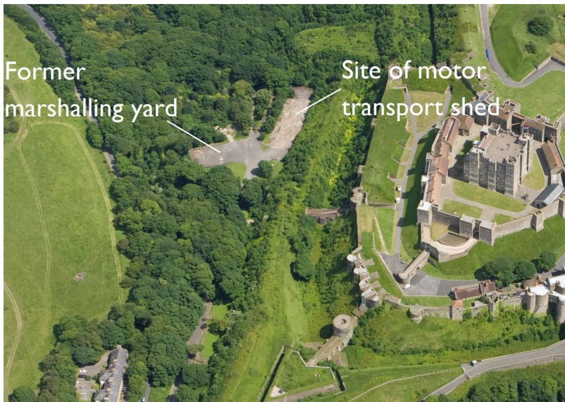
Figure 7. Aerial view of northern end of Broadlees Bottom, with two car parking areas highlighted.
