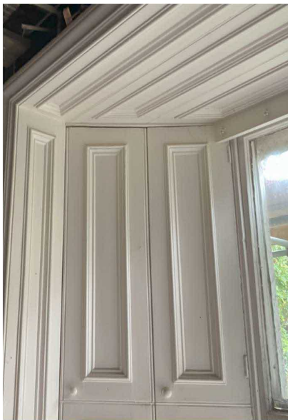
Wood panelling and shutters around windows and doors at rear of ground floor.
