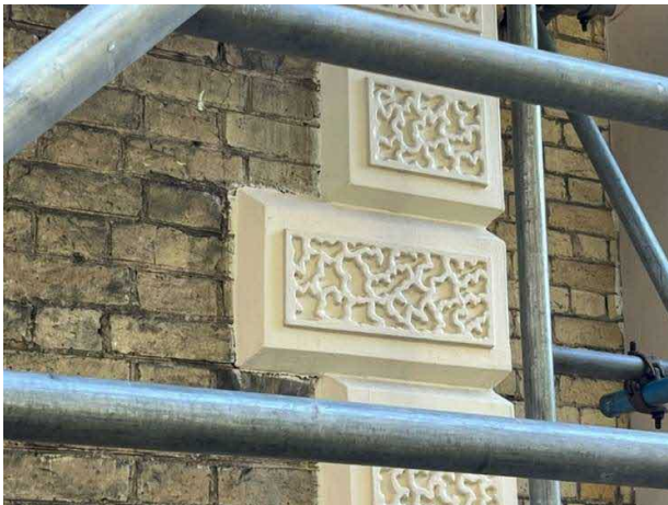
Detailed stone sets to corner returns.
