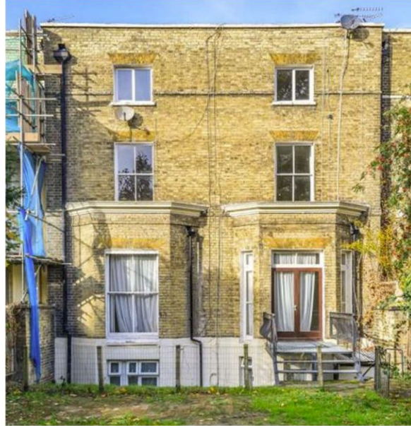
No. 3 South Terrace (rear).
