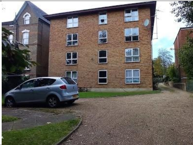
Photograph 1: Eastern elevation of the building.
