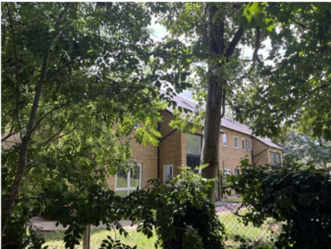
Plate 6 View of development immediately to the south of the site incorporating two storeys plus attic. Granted planning permission in 2007 (ref 07/03230/P).
