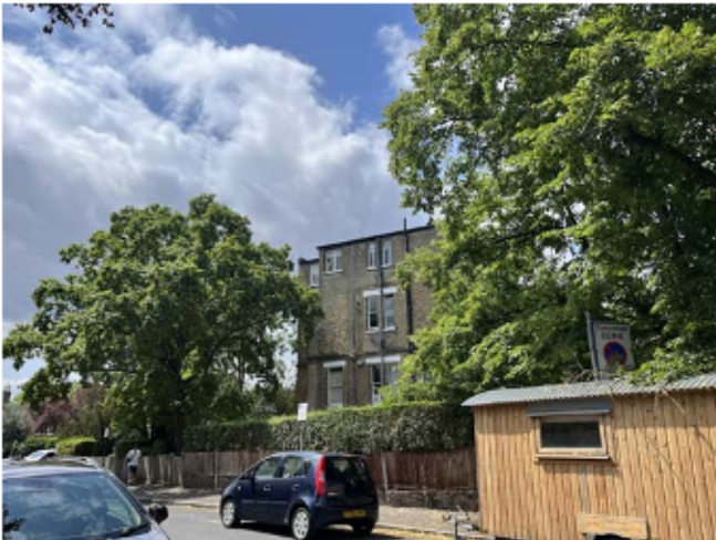
Plate 12 View showing flat roof of historic property south west of the site.
