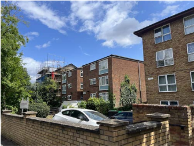
Plate 9 View of the site (right) and Ashleigh Lodge, left/centre.
