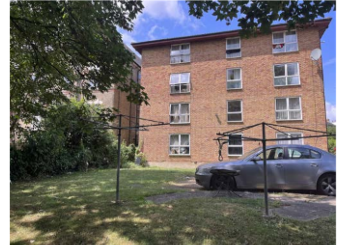
Plate 5 View of rear elevation of The Hawthorns.
