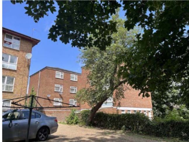
Plate 4 View looking north west towards Ashleigh Lodge from rear garden, note, this development projects further east than the historic rear building line.
