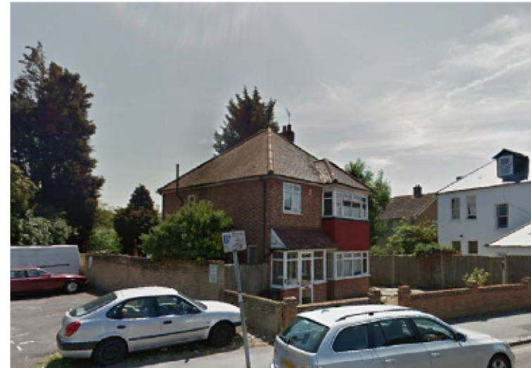
Plate 16 View of previous hipped roof property at 282 Holmesdale Road pre 2017.
