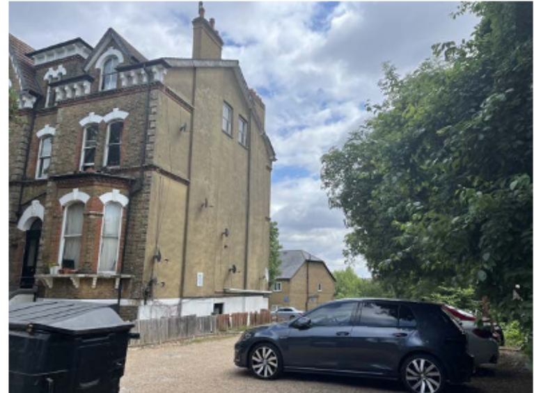
Plate 22 View showing No. 61 Warminster Road, locally listed and its relationship with the development consented in 2007.
