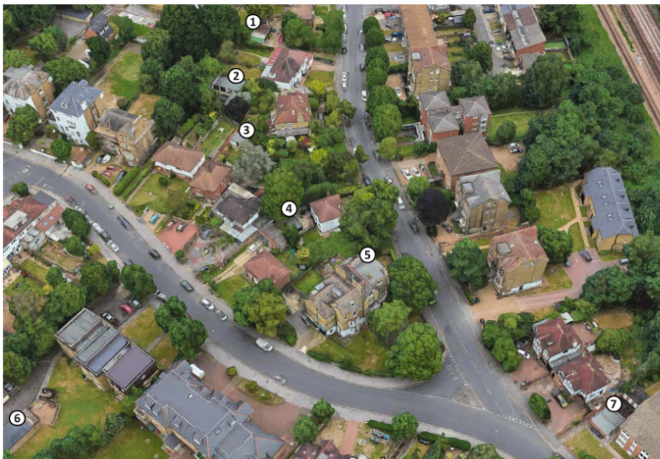
Figure 11 Showing buildings with flat roofs within the Lancaster and Warminster Road character area.
