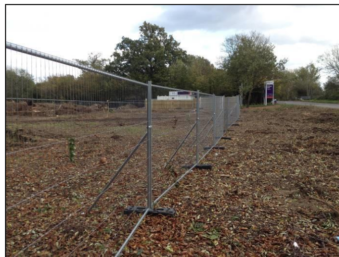
On site examples of appropriate tree protection fencing installed as recommended within BS5837
