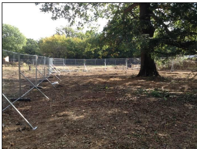
On site examples of appropriate tree protection fencing installed as recommended within BS5837
