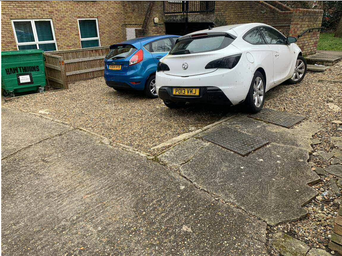
Photo 6: | Manhole covers in front garden
