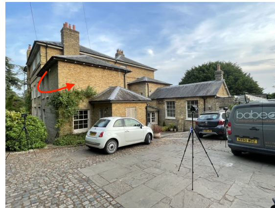
Roost B | 76 common pipistrelles emerged from a gap in the eaves on the eastern elevation of the property.
