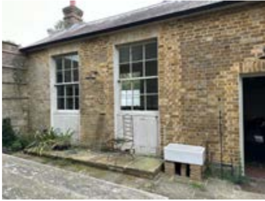
Fig 12, current view of the western mission room wall overlooking the garden. The areas of lighter brick and modern cement pointing indicates much rebuilding
