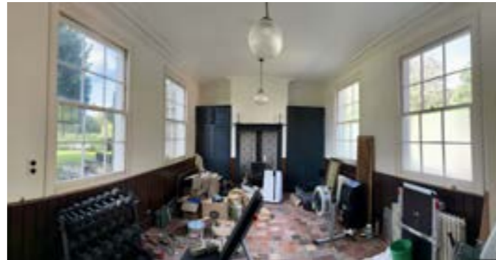
Fig 9, current interior view, with 1990s fenestration
