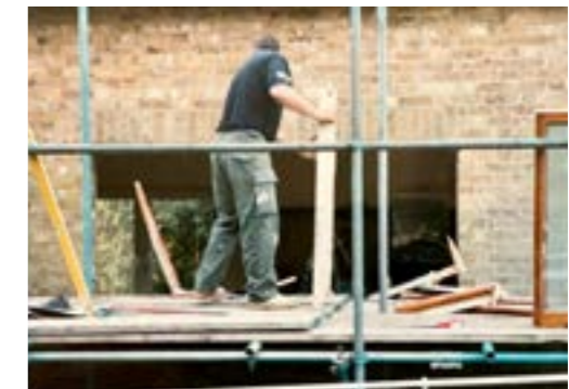
Fig 6 casement window being removed c.1995
