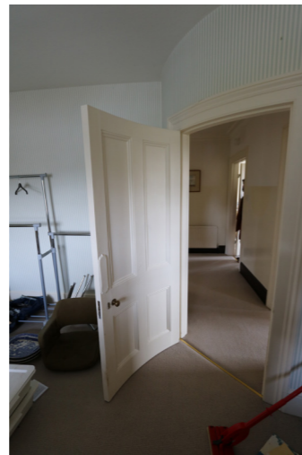
2. Existing curved door on second floor level.
