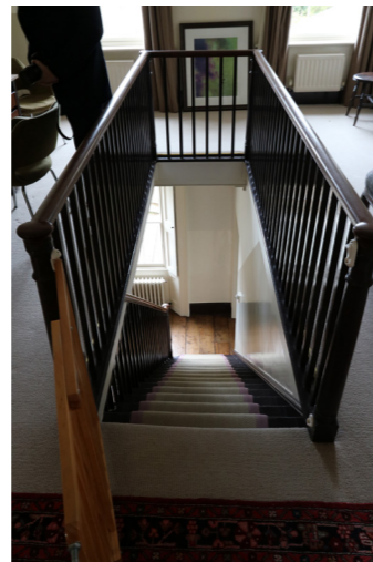
1. Existing secondary stair on second floor level
