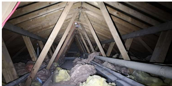
Internal view showing timber frame structure.
