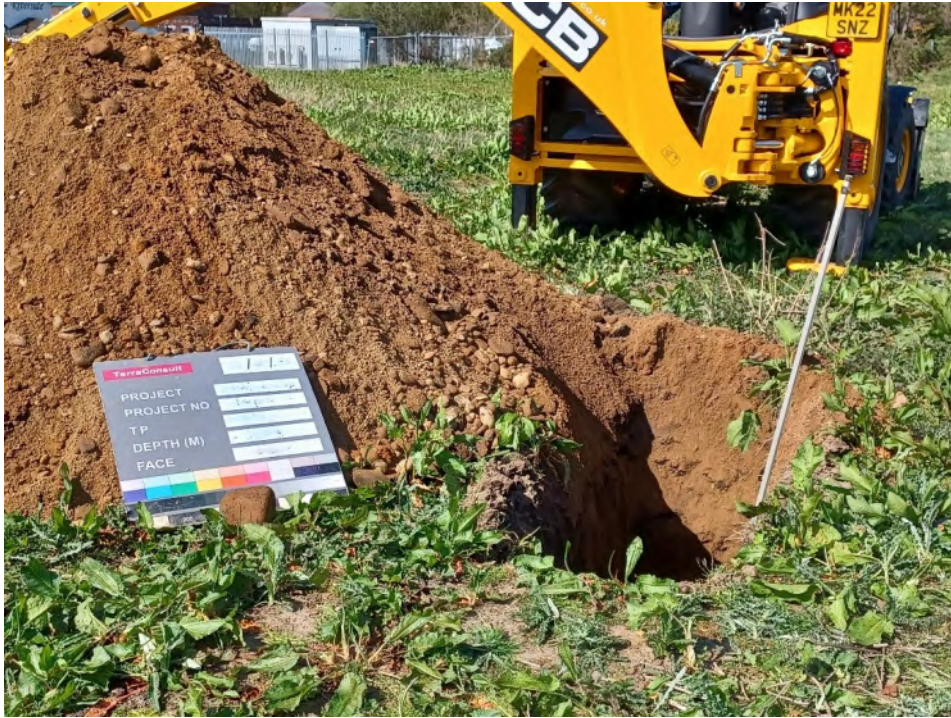
TP06 Trial pit and spoil heap.
