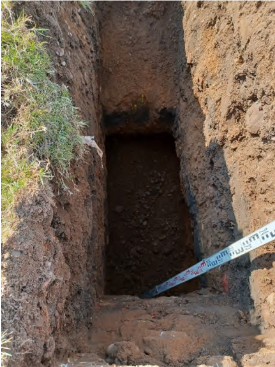
TP13 Base of pit.
