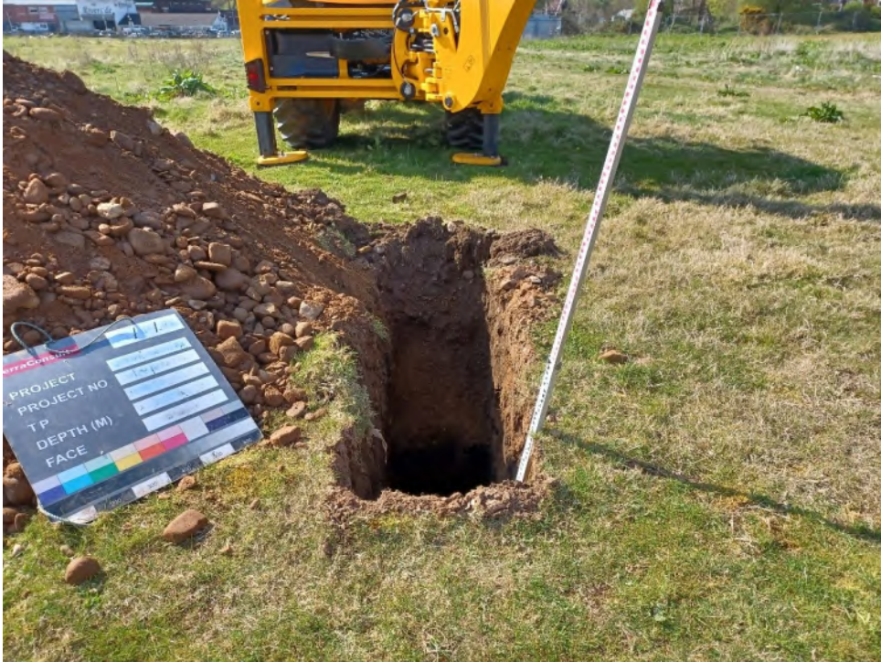
TP13 Face C and spoil.
