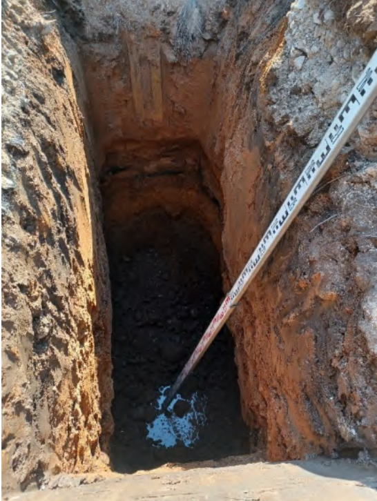
TP01 Base of pit.
