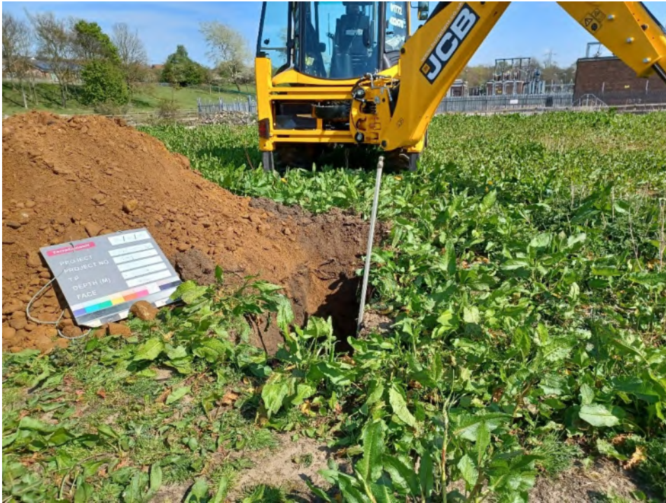
TP09 Trial pit and spoil heap.
