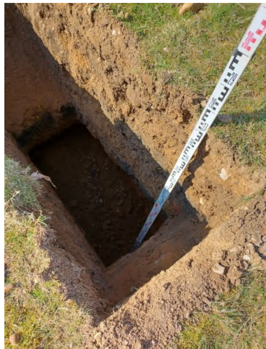
TP13 Base of pit.
