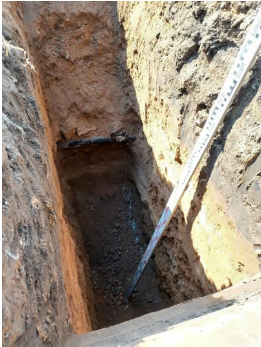
TP12 Face B, C and black polyethene pipe (land drain).
