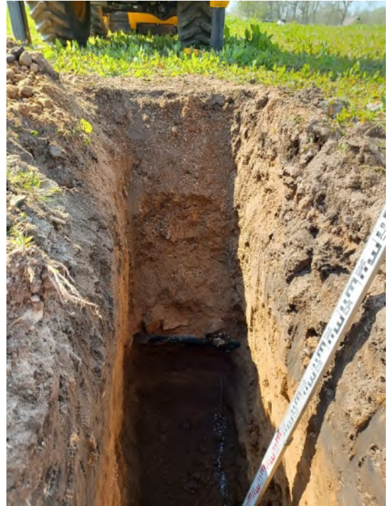
TP12 Face C and black polyethene pipe (land drain).
