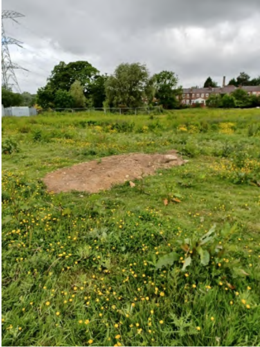
SA01 After backfill.
