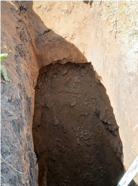
TP06 Base of pit and collapse.
