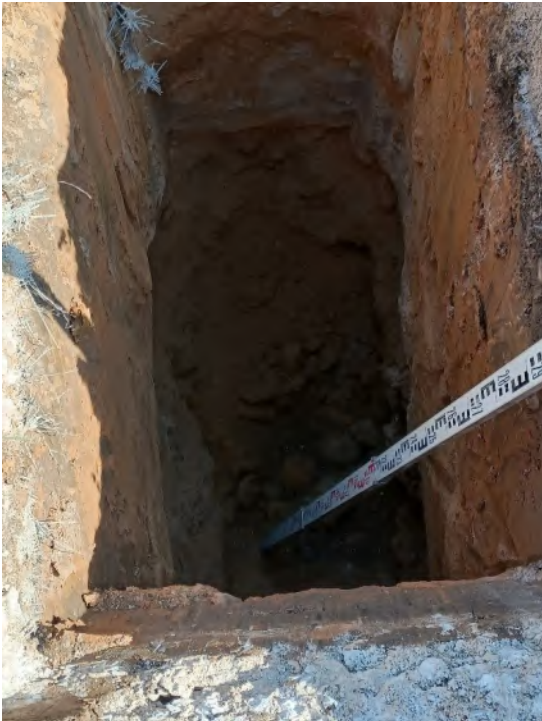
TP04 Base of pit.
