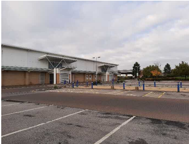
Photo 1: The site, as viewed from the car park to the east
