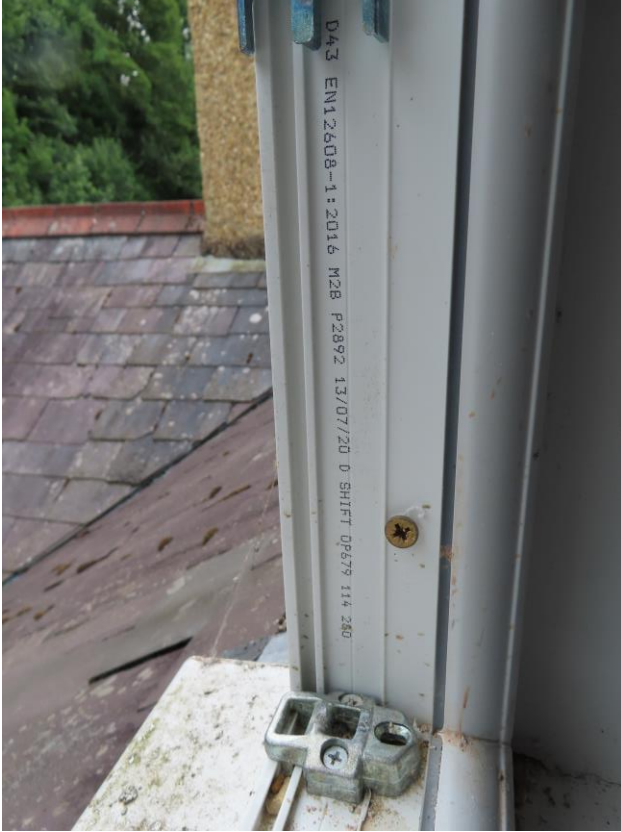
Typical Existing Second Floor Frame
