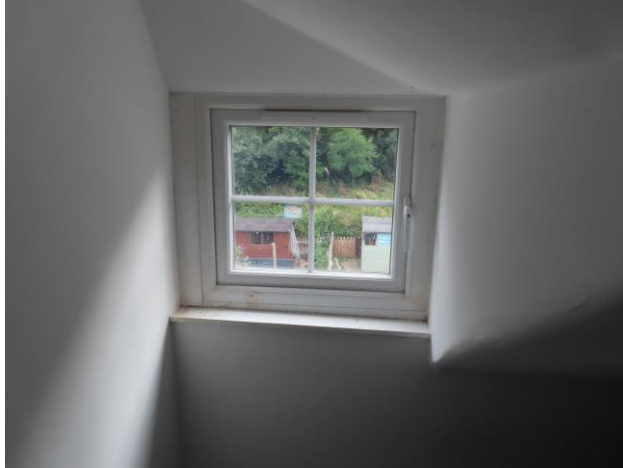
Second Floor Rear Window
