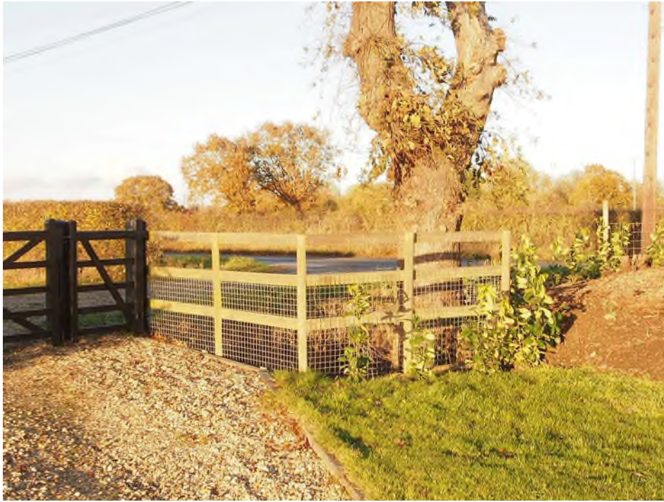
View of existing entrance gate
