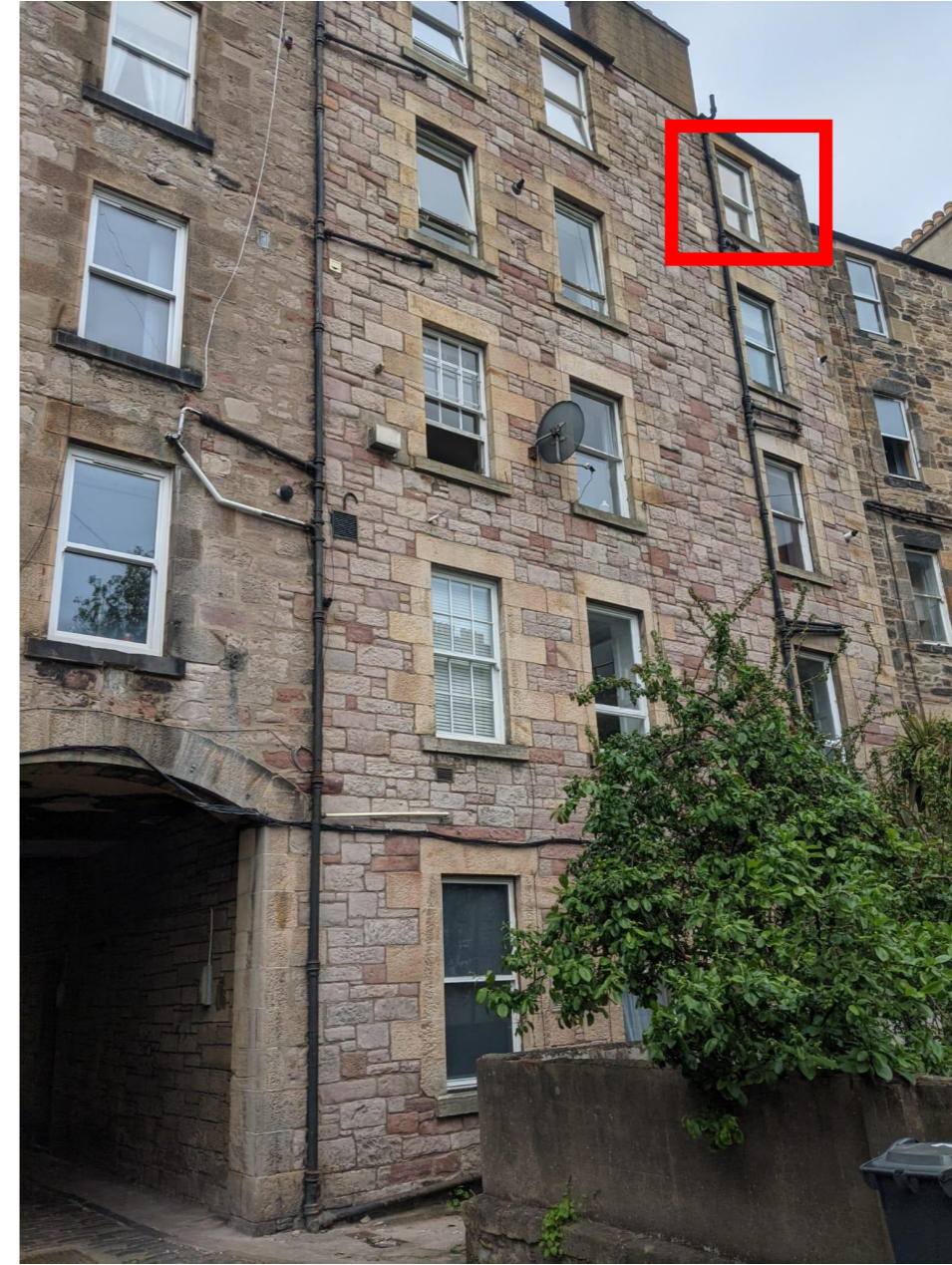
Rear view after window replacement. (New window highlighted).
