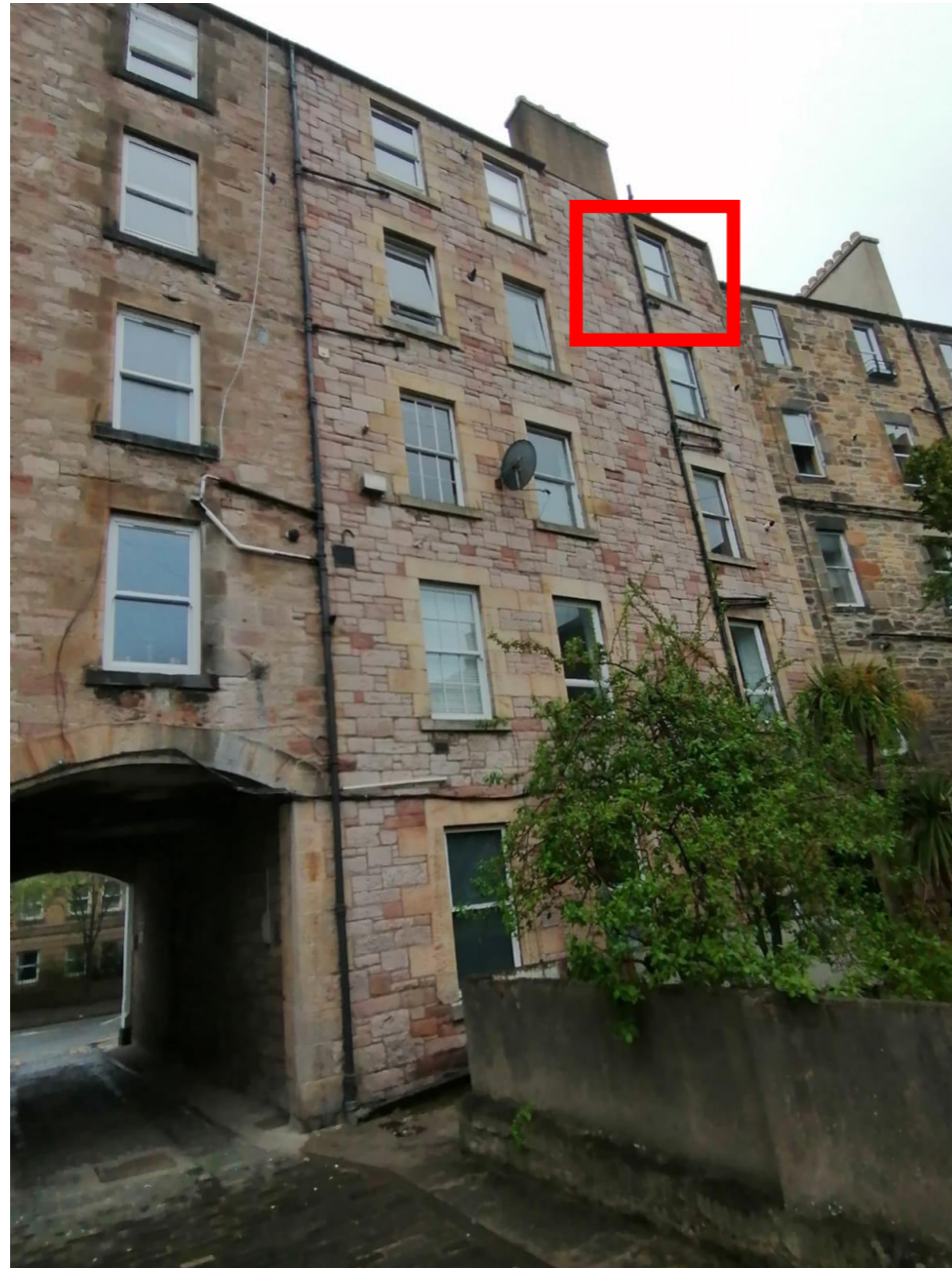
Rear view prior to window replacement. (Affected window highlighted).
