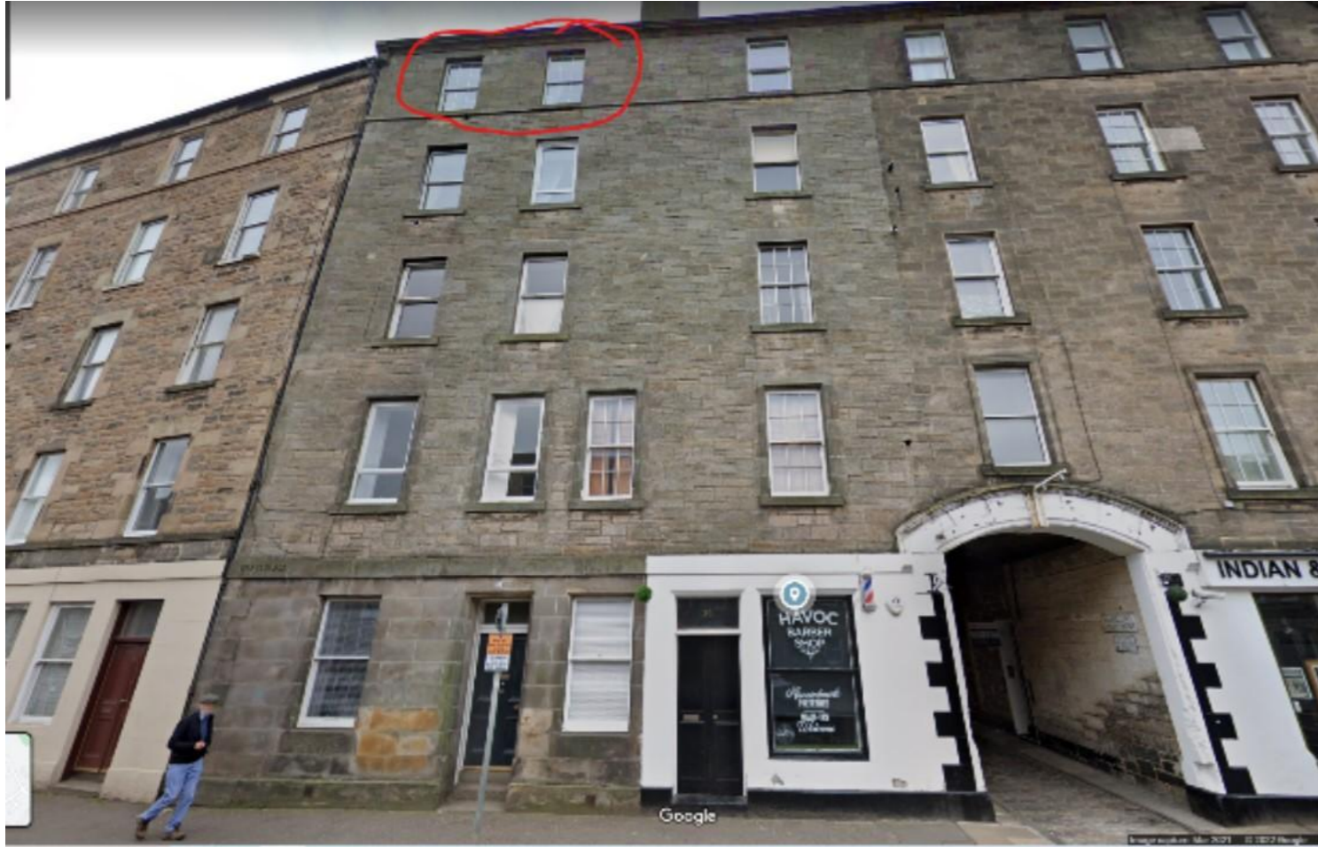
Street view prior to window replacement. (Affected windows highlighted).
