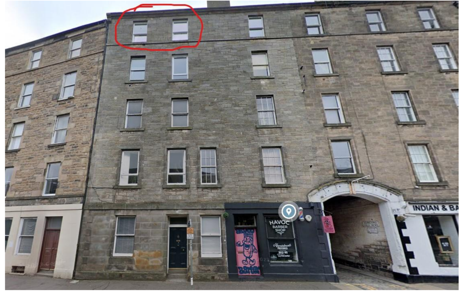
Street view after window replacement. (New windows highlighted).
