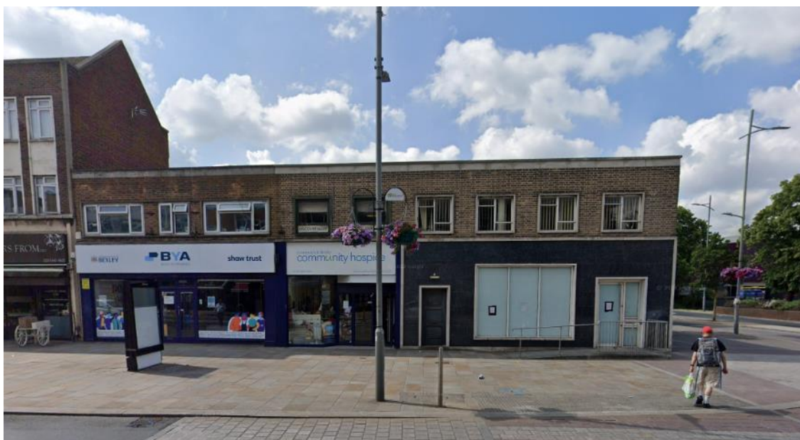
Site in street scene
