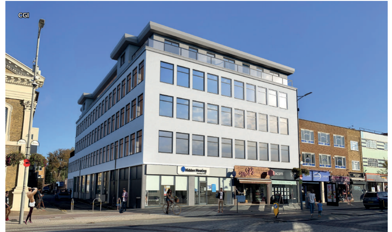
210-214 Broadway as completed
