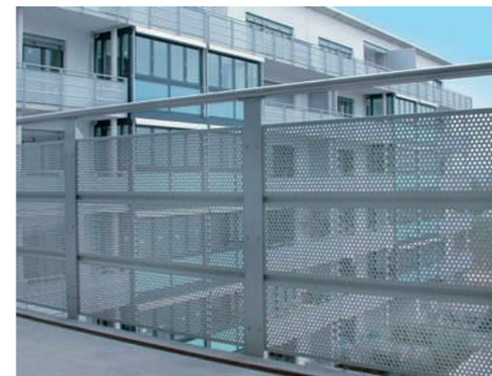
Metal framed balustrade with mesh infill panels
