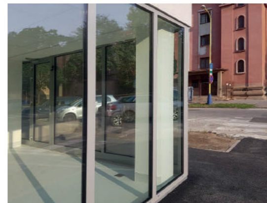
Metal framed double glazed windows
