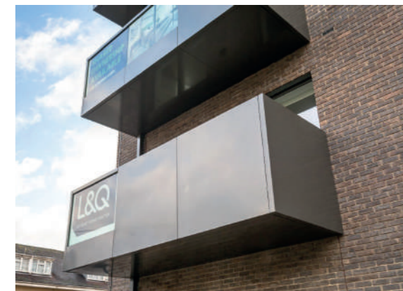
Solid balustrades to rear elevation
