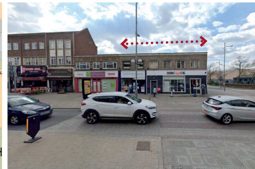
Front elevation of 235 & 237 Broadway
