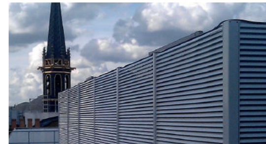
Metal louvre enclosure to roof top plant
