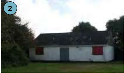
THE EXISTING CSM CHANGING / FACILITIES BUILDING
