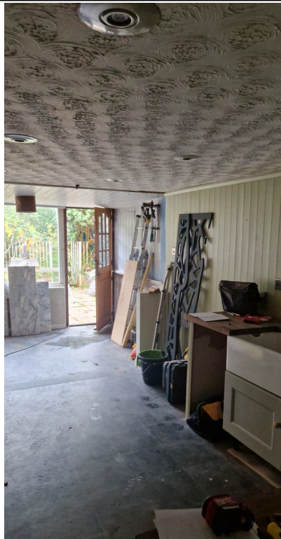
Internal (kitchen, looking towards garden). Note artex ceiling and shiplap cladding.
