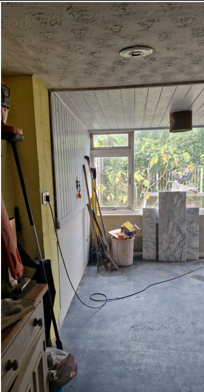
Internal (kitchen, looking towards garden). Note artex ceiling and shiplap cladding.
