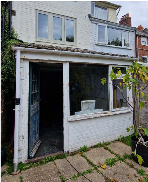
South (rear showing existing extension)
