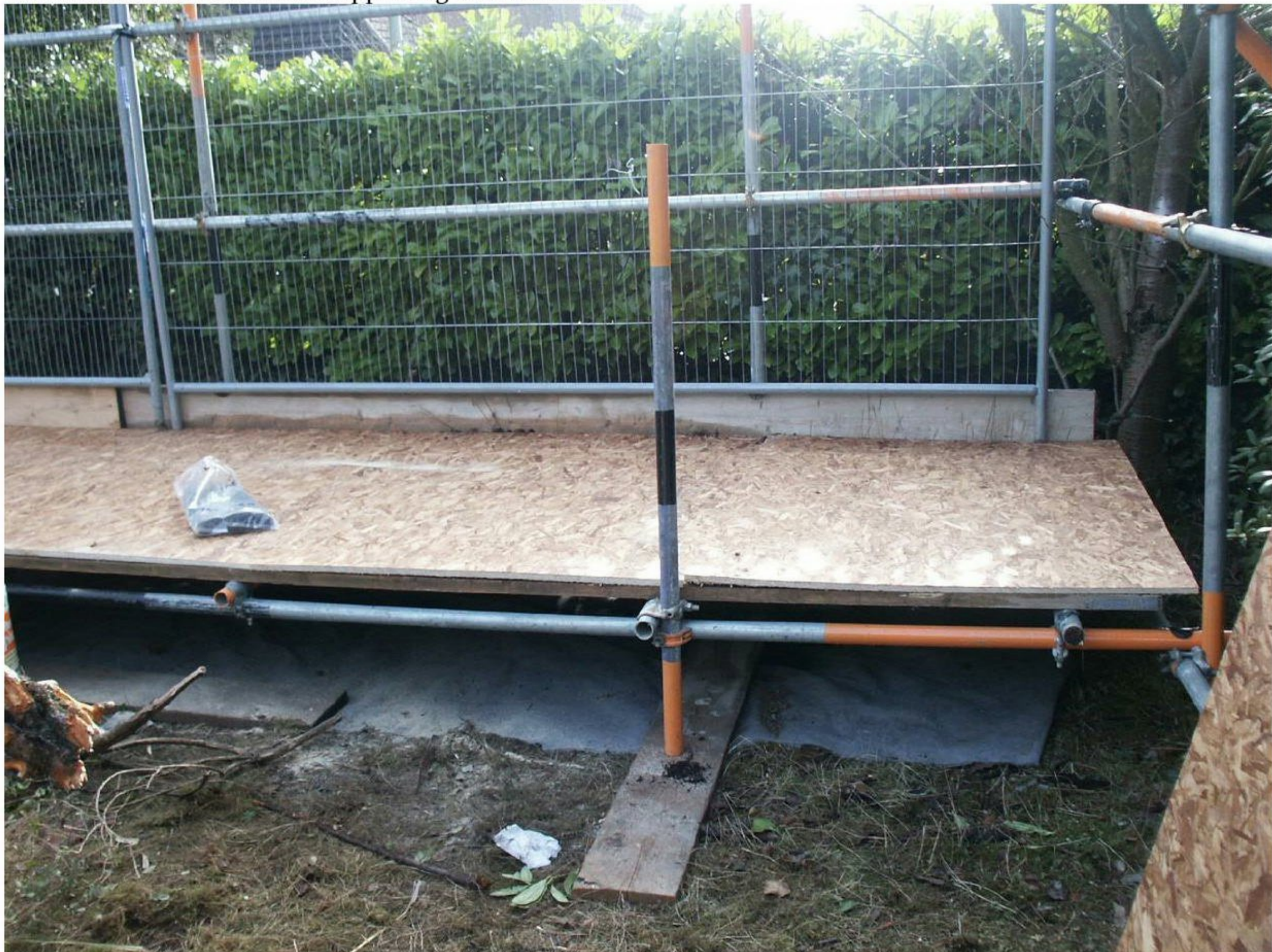
Photo 2 Scaffold framework supporting wooden boards
