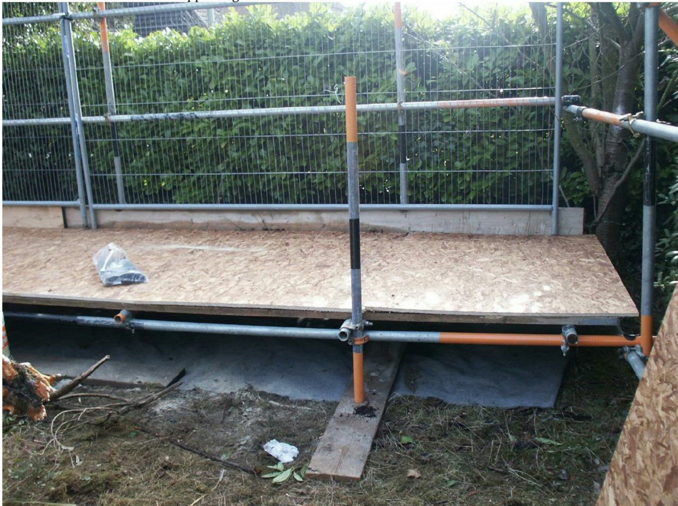
Photo 2 Scaffold framework supporting wooden boards
