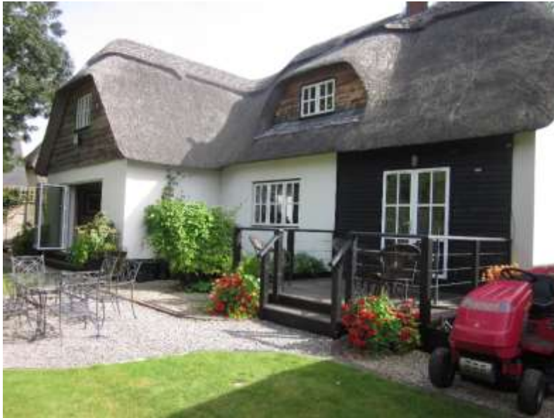
Rear of Weir Cottage
